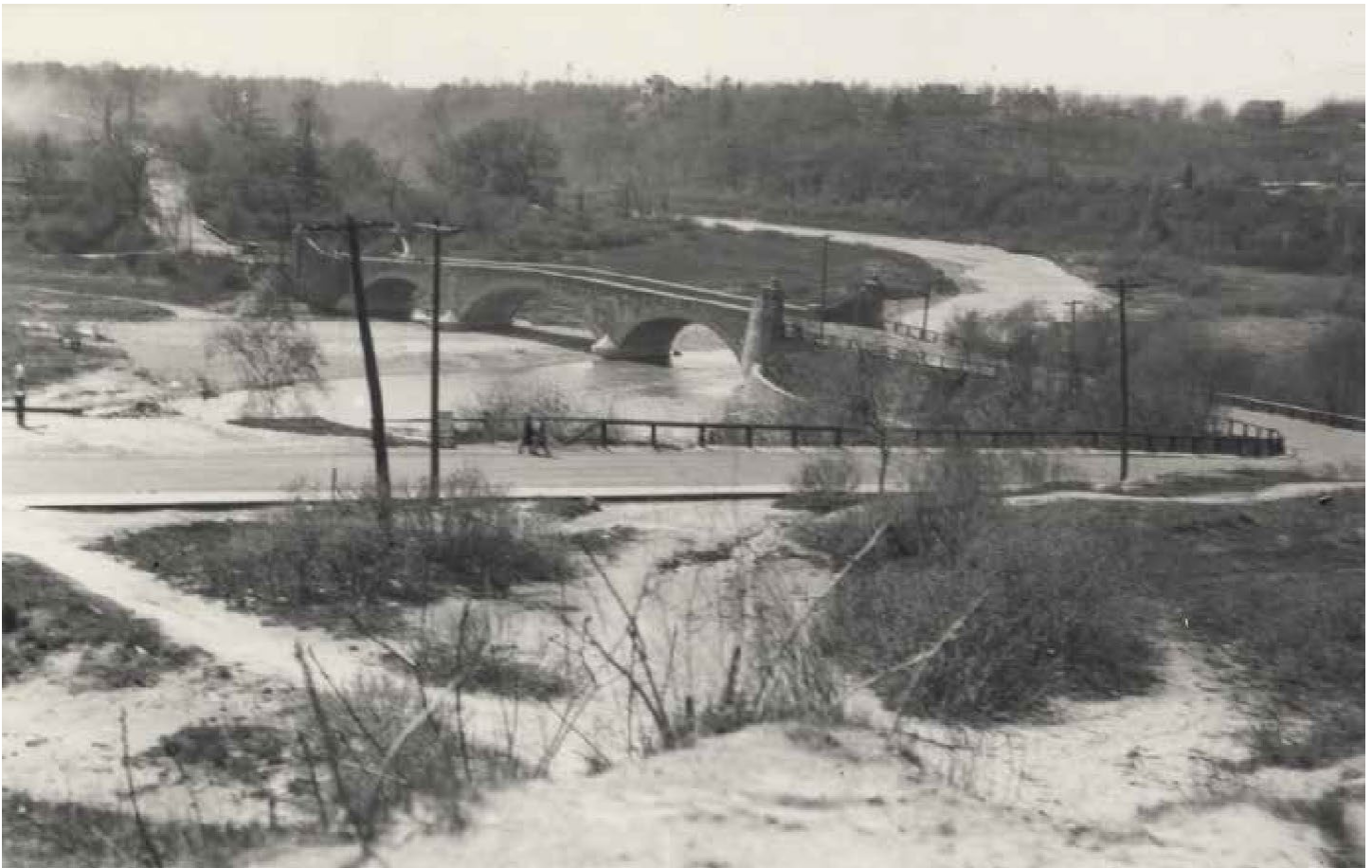
Figure 22: Old Mill Rd., looking west to bridge (built 1916) across Humber River. Viewed between Catherine Street & Old Mill Road
