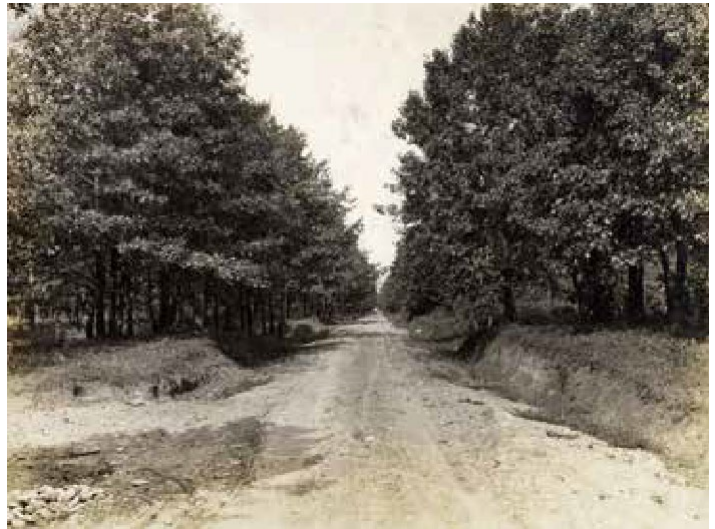
Figure 18: Construction of Baby Point Road
