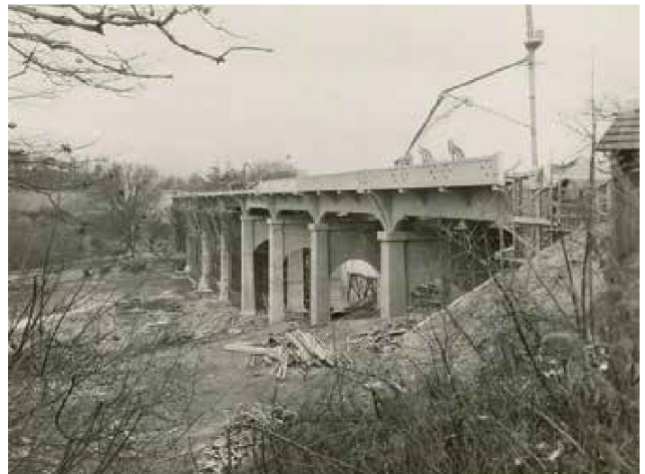
Figure 23: Dundas Street West, bridge over Humber River looking east, during construction, 1928 (Toronto Public Library)
