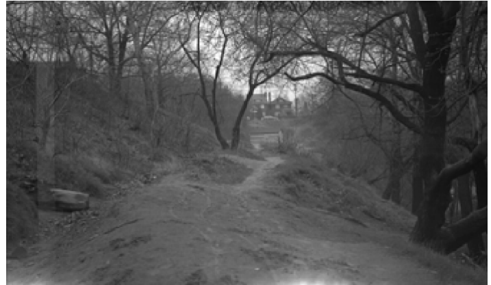
Figure 11: Remnants of Belt Line Railway. G.T.R. Belt Line, looking north from north of Humberview Rd. to Methuen Ave., east of Humbercrest Blvd., Toronto, Ont. 1953 (Toronto Public Library Digital Archives)
