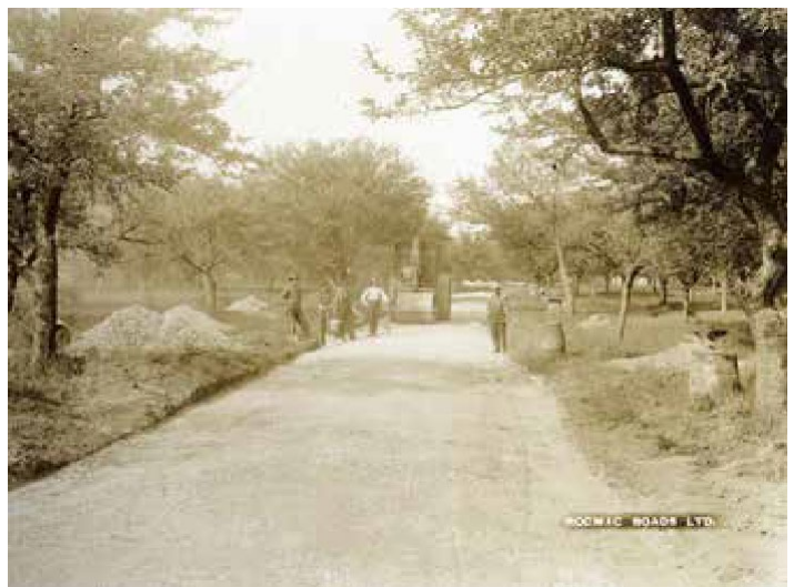
Figure 19: Construction of Baby Point Road (2)
