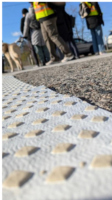
FINCH CORRIDOR TRAIL MID-BLOCK INTERSECTION – TESTING DIRECTIONAL TWSI
