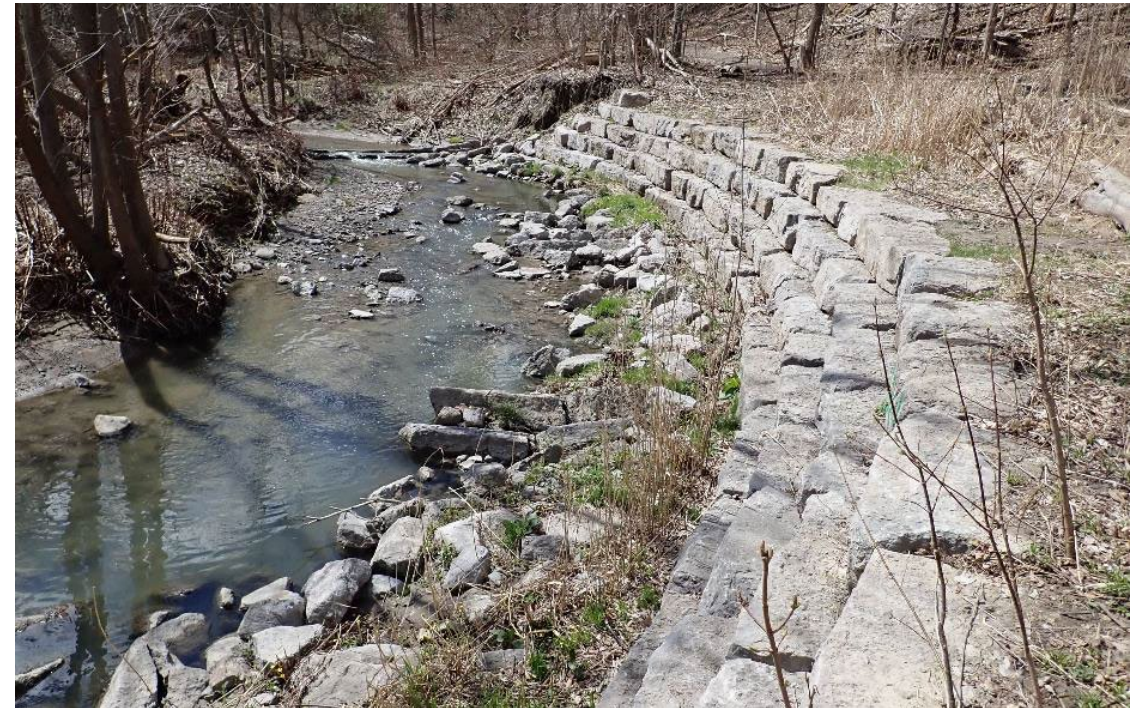
Photo of an armourstone bank and vegetated stone treatment at the water's edge along the stream bank of Burke Brook.
