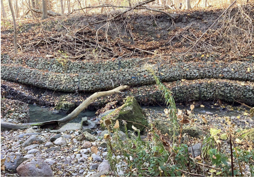
Photo 3 - November 20 th , 2023 – Example of failed (5) gabion baskets.
