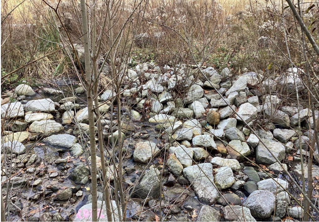
Photo 9 - November 20 th , 2023 – Example of failed (5) vegetated rock buttress. Most of the rip rap is displaced.
