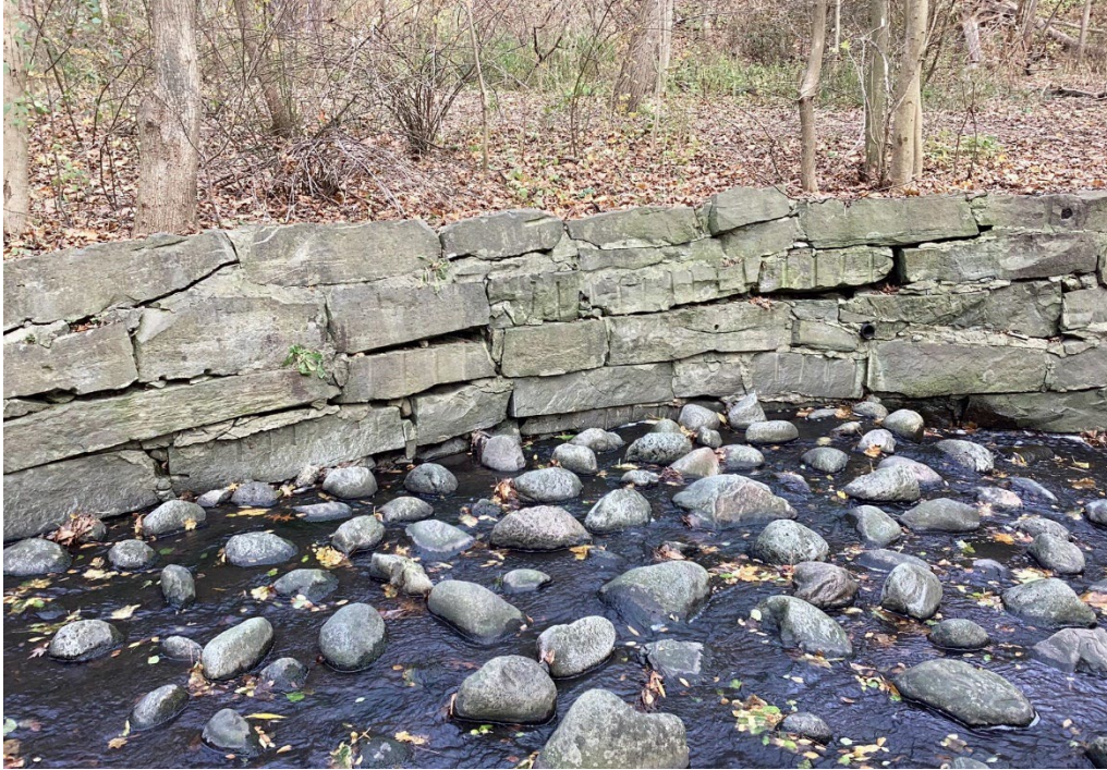
Photo 5 - November 20 th , 2023 – Example of poor (3) quarried block wall. Misaligned and cracked stones visible.
