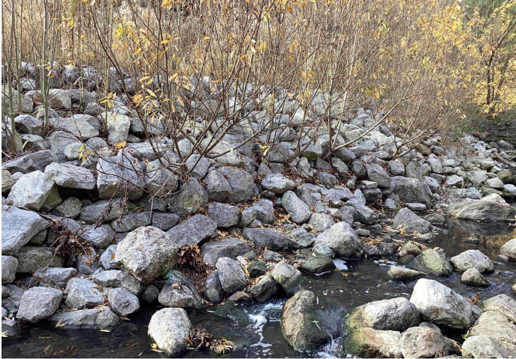
Photo 7 - November 20 th , 2023 – Example of poor (3) rip rap revetment. Displaced rip-rap visible in the channel.
