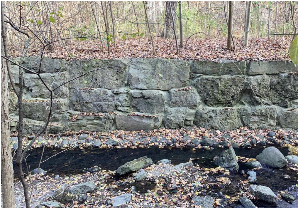
Photo 4 - November 20 th , 2023 – Example of good (1) quarried block wall.
