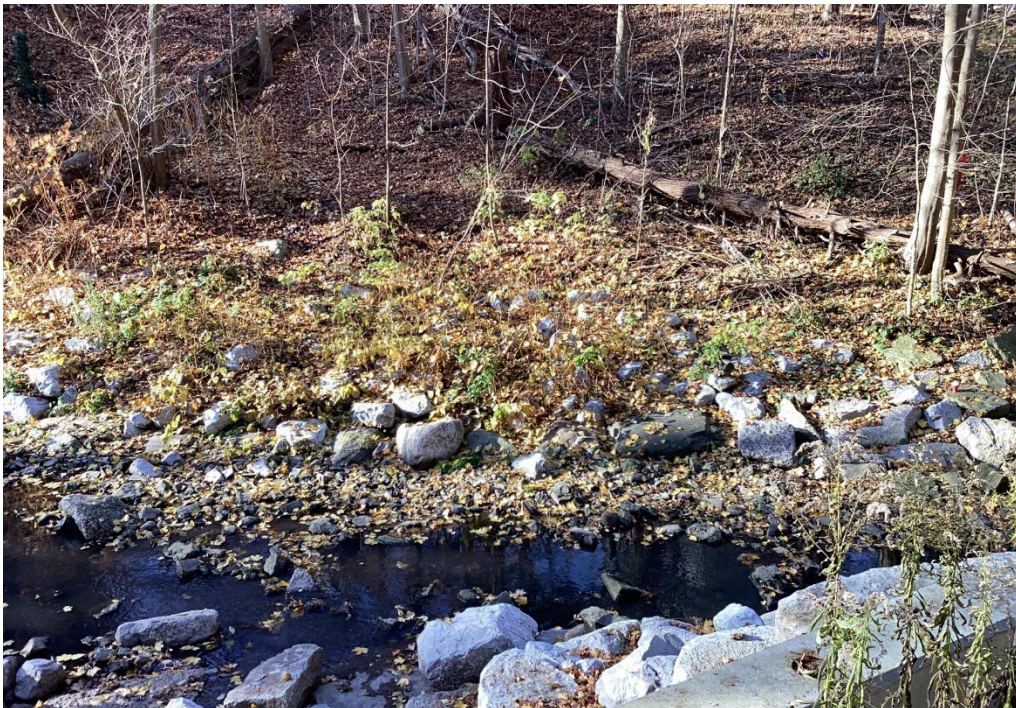
Photo 8 - November 20 th , 2023 – Example of fair (2) vegetated rock buttress.
