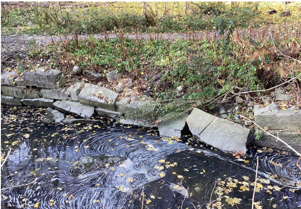
Photo 6 - November 20 th , 2023 – Example of failed (5) quarried block wall.
