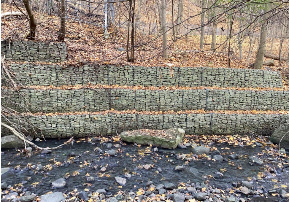
Photo 1 - November 20 th , 2023 – Example of fair (2) gabion baskets. Some undermining visible.
