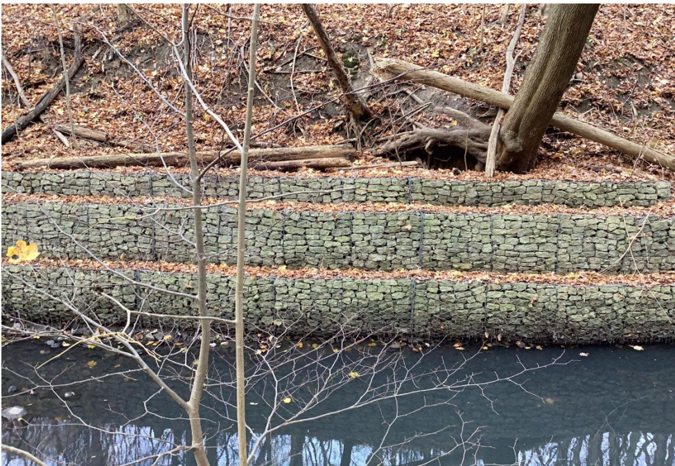
Photo 2 - November 20 th , 2023 – Example of poor (3) gabion baskets. Slightly slumping and undermining visible.
