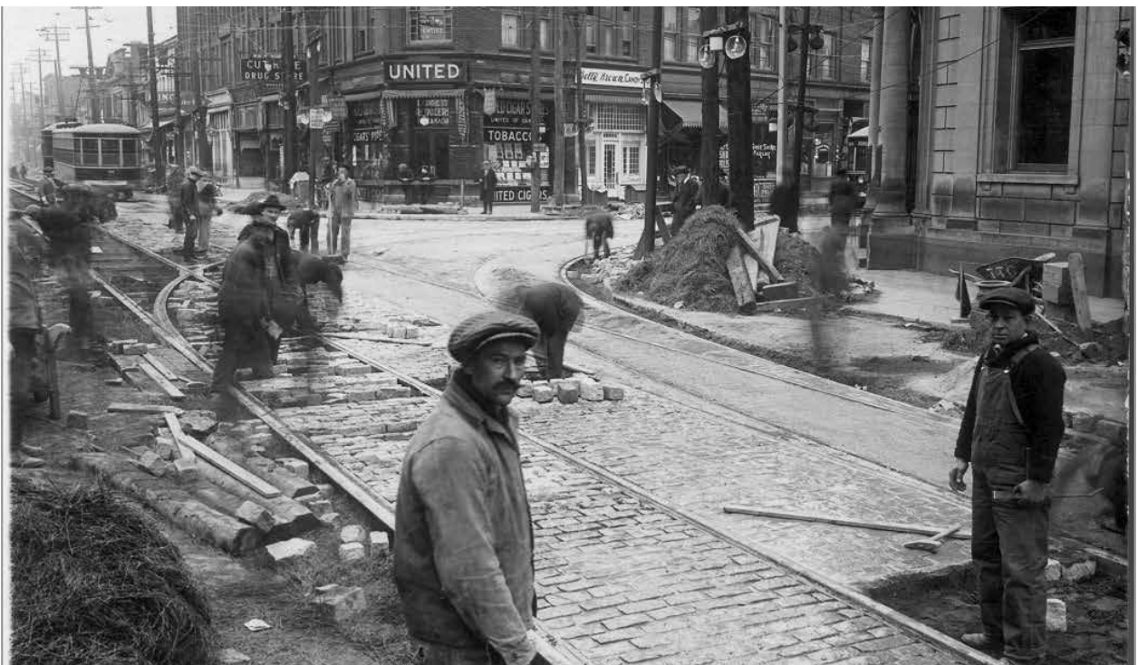
Figure 50: Laying streetcar tracks at the corner of Dundas Street West and Keele Street, November 1923 (City of Toronto Archives: Fonds 16, Series 71, Item 2815).
