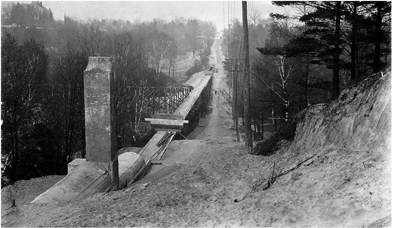
Figure 47: The height of the sewer grate shows how significantly Bloor Street's grade was raised in 1914. ( City of Toronto Archives: Series 1231, Item 1201 ).
