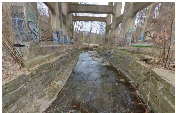
Photo 3.12 Facing north. CP railway bridge crossing.
