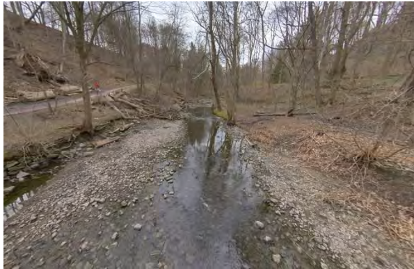
Photo 2.11 Facing northwest. Unarmoured section of channel.
