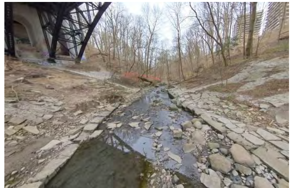
Photo 1.10 Facing south. Armourstone and shale tile line banks through St Clair bridge crossing. Debris from slope failure visible in left side of photo.
