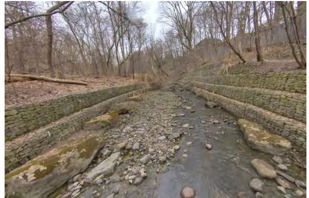
Photo 1.4 Facing north. Gabion baskets stable on both banks.
