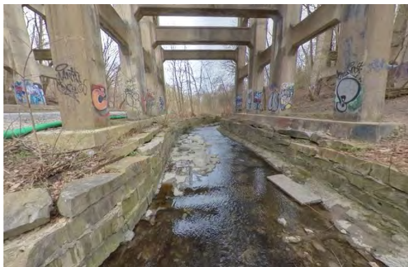
Photo 3.11 Facing south. CP railway bridge crossing.
