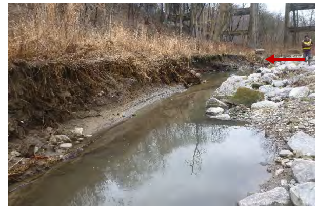
Photo 3.10 Facing downstream. Erosion on left bank. Stormwater outfall channel connects to main channel at red arrow.
