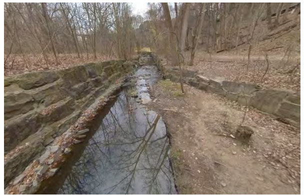
Photo 3.4 Facing south. Watermain crossing location.
