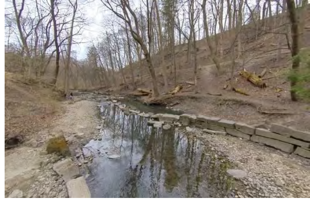
Photo 2.10 Facing south. Channel has widened beyond historical banks, leaving armourstone in the middle of channel.
