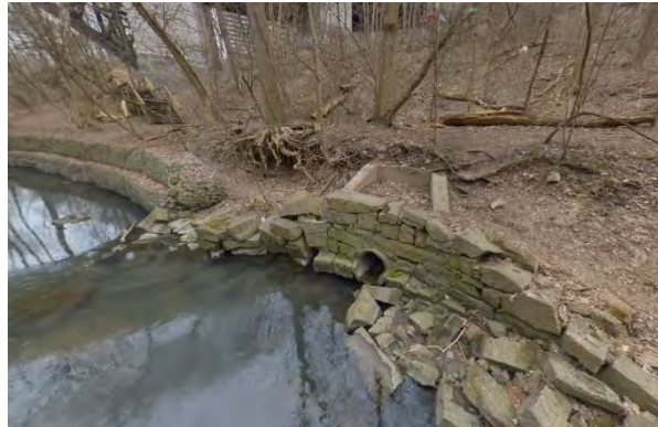
Photo 1.7 Facing south. Outflanked stormwater outfall OF3862313685 on right bank. Evidence of scour on bank above outfall.
