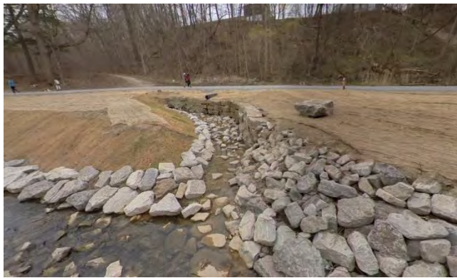
Photo 3.9 Facing east. Rosehill pumping station storm outfall channel, 2023.
