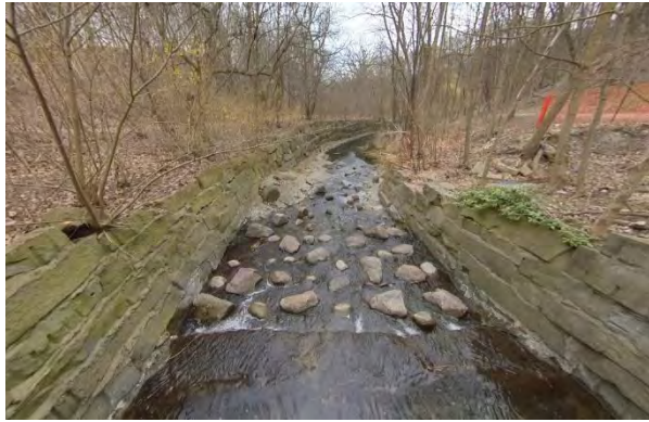
Photo 3.1 Facing south. Concrete apron spillway downstream of pedestrian crossing.
