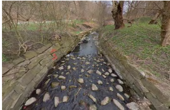
Photo 4.5 Facing south. Concrete grade control apron.
