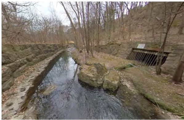
Photo 3.3 Facing south. Rosehill reservoir discharge outfall OF800169 on right bank.
