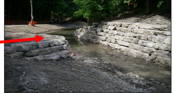
Taylor-Massey Creek maintenance hole stabilized and protected behind armourstone
