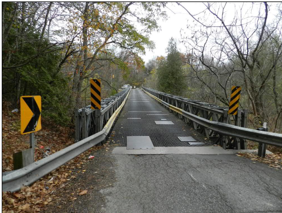
View Looking South (Note Plate Repairs to Deck)
