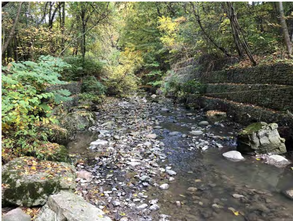
Photo 12 October 28, 2020. M1, facing upstream.
