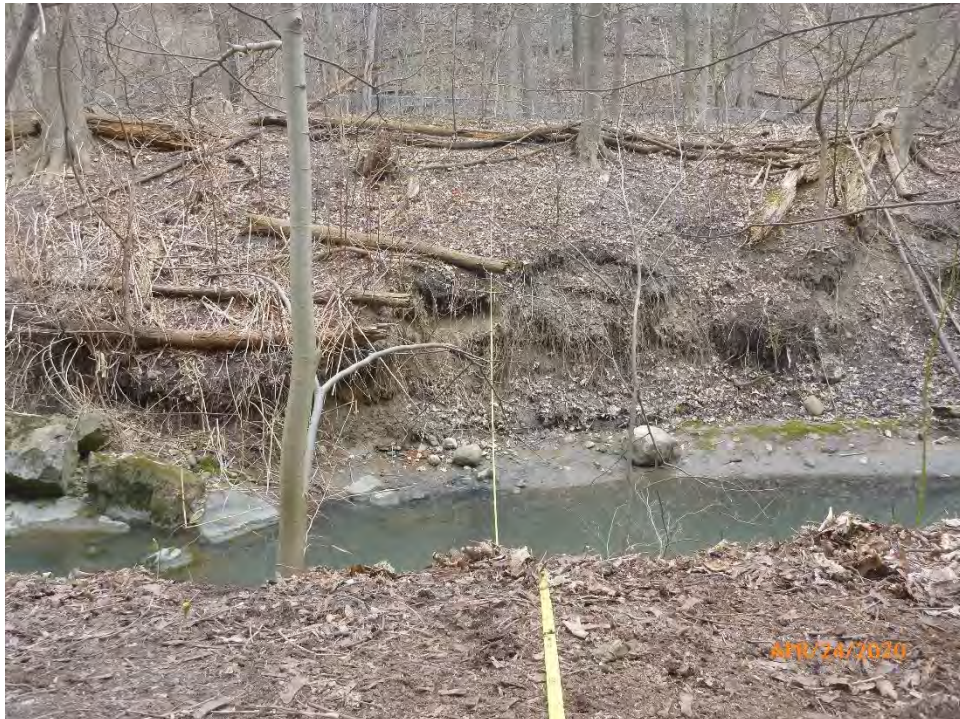
Photo 26 April 24, 2020. M2, east bank.
