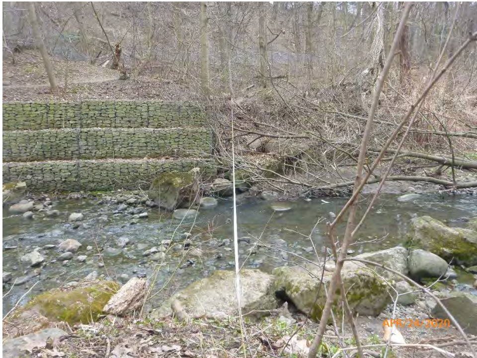
Photo 6 April 24, 2020. M1, east bank.
