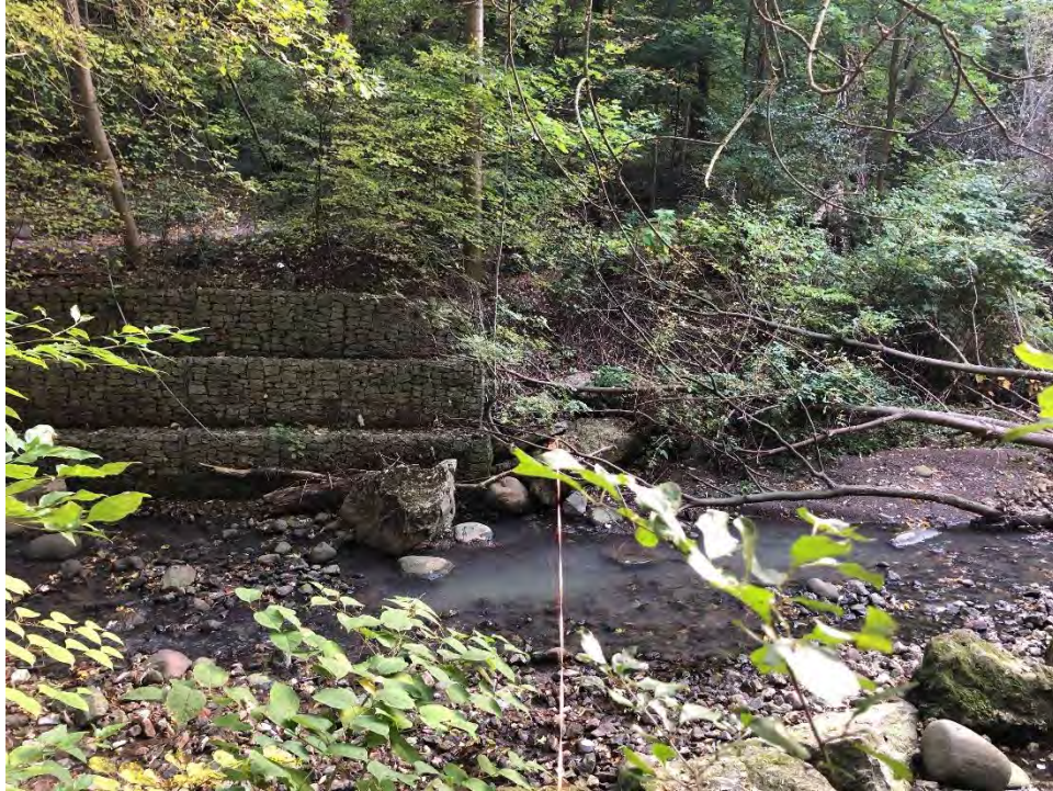
Photo 9 October 20, 2021. M1, east bank.
