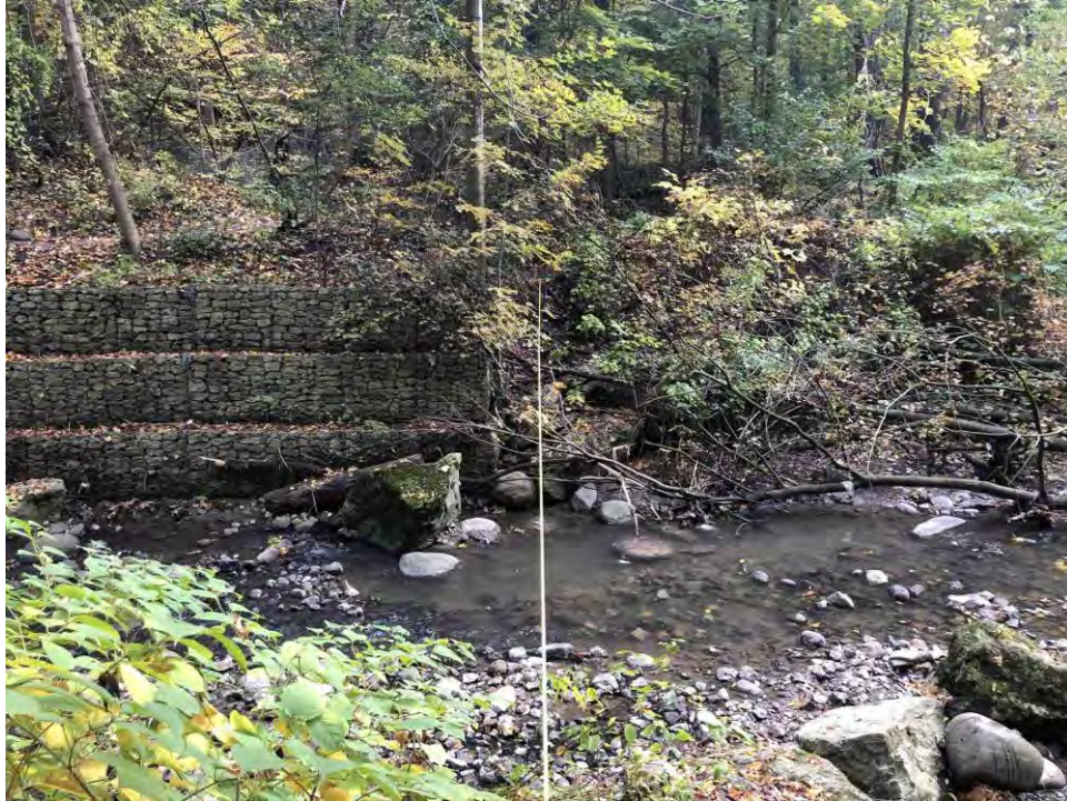
Photo 7 October 28, 2020. M1, east bank.
