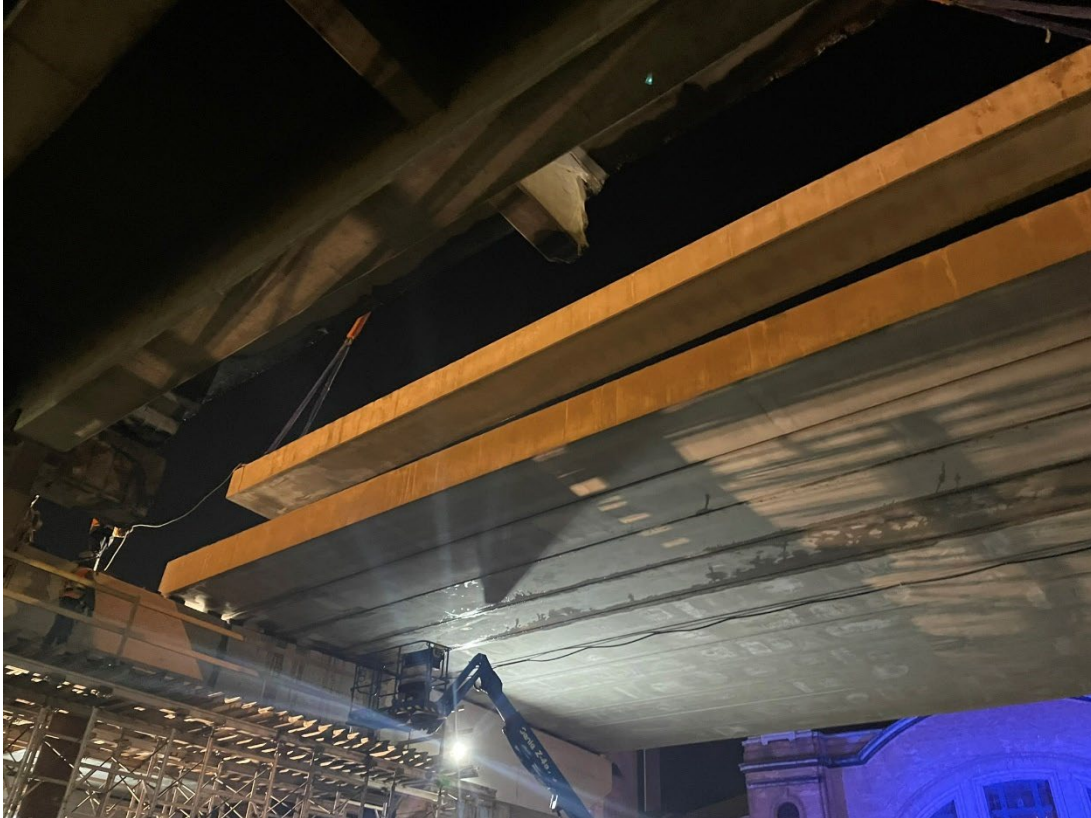
New girders being installed.
