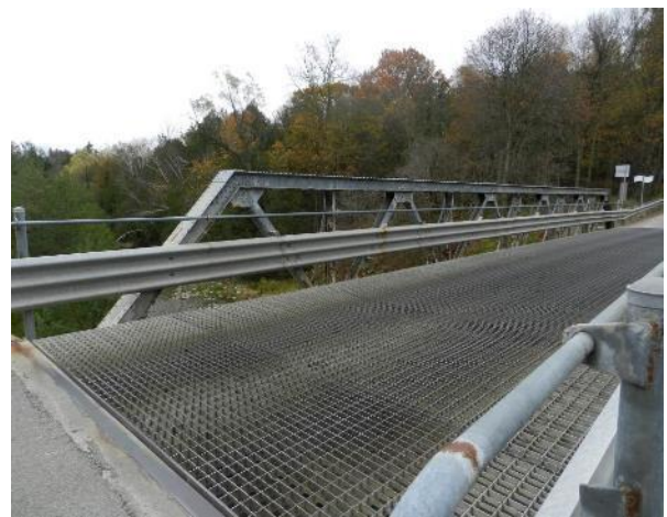
Figure 29: Hillside Bridge Deck, Guide Rail and Railing
