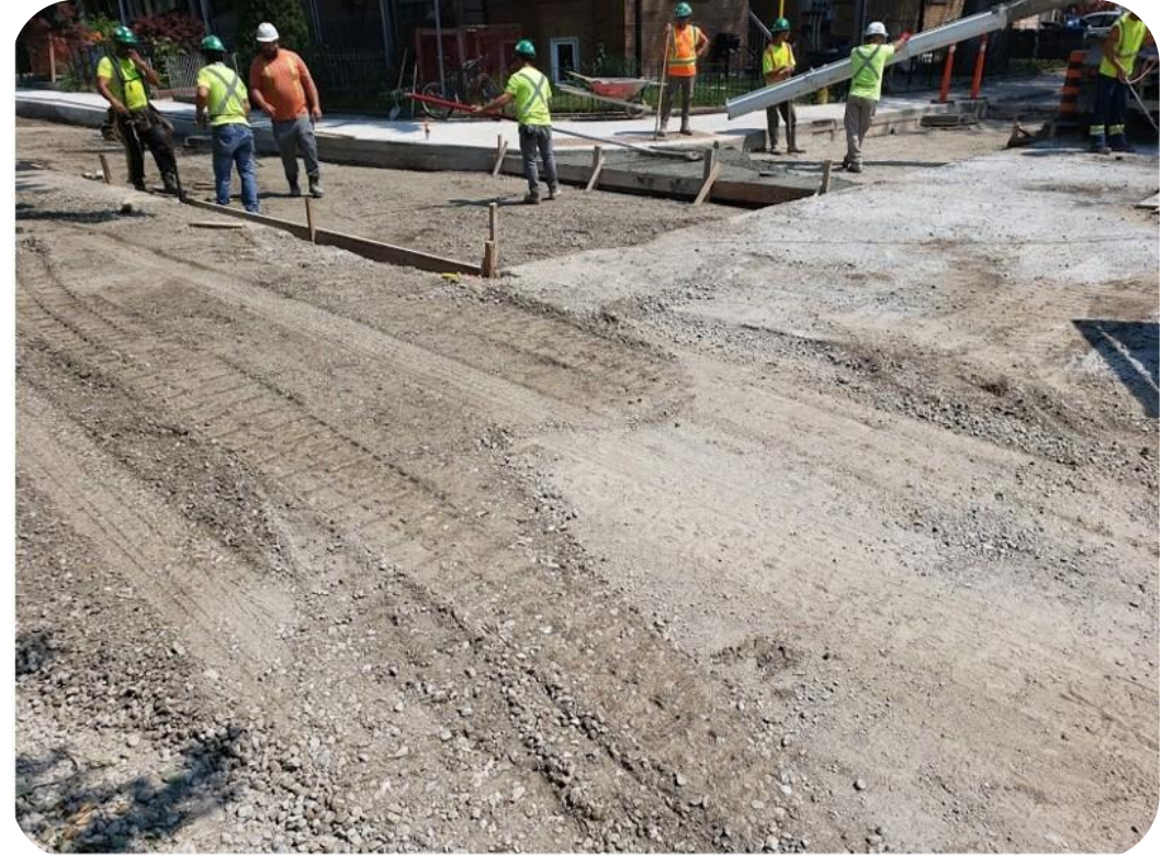
Example of road reconstruction
