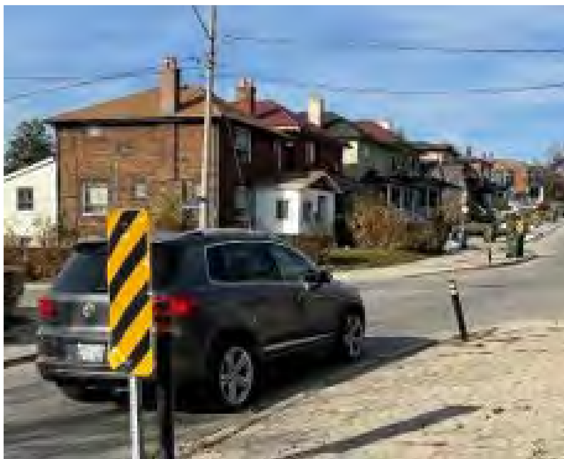
Curb extension with concrete and asphalt and signage
