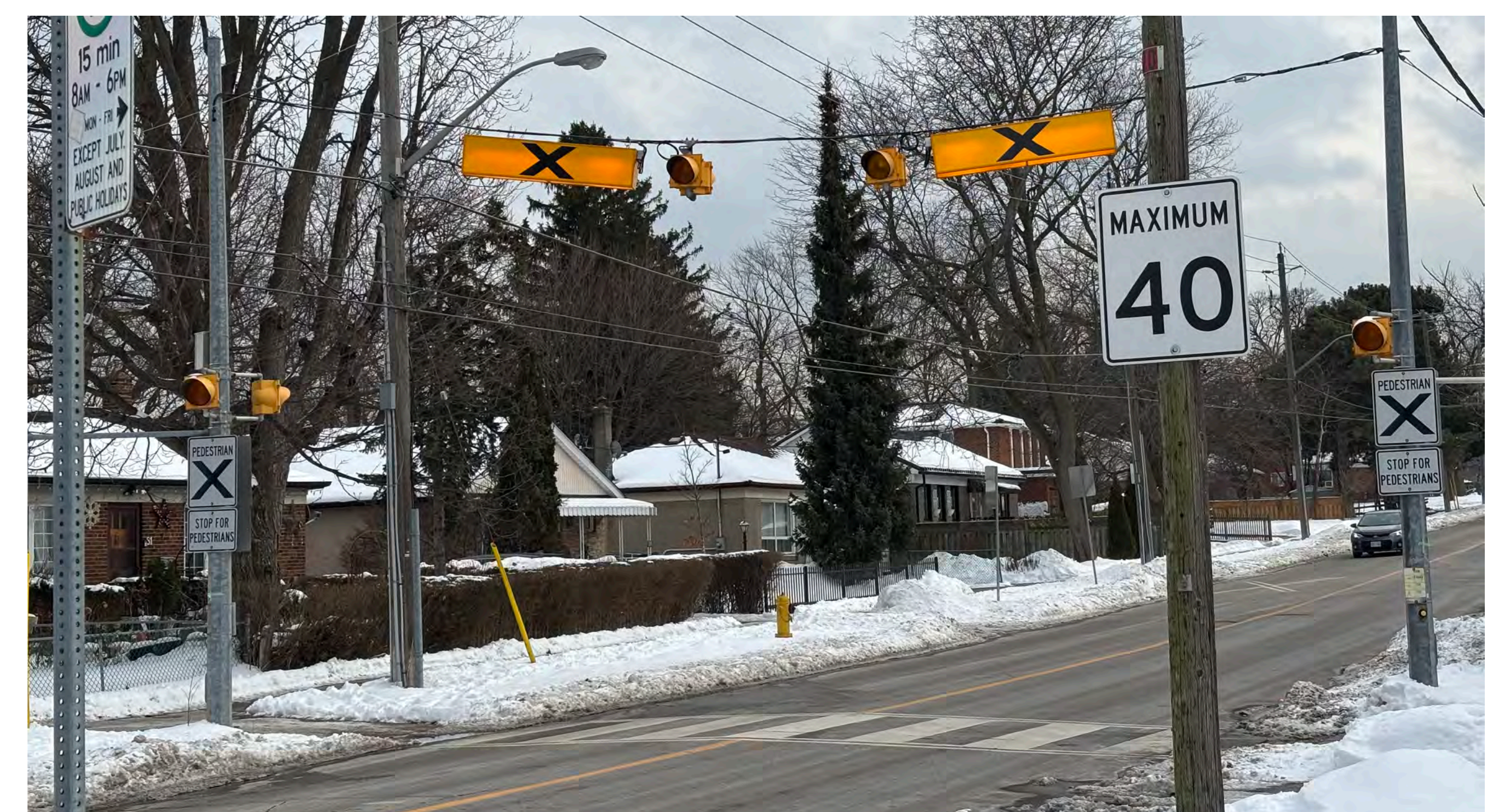
Flashing Beacon Installed on Mason Rd In the School Safety Zone
