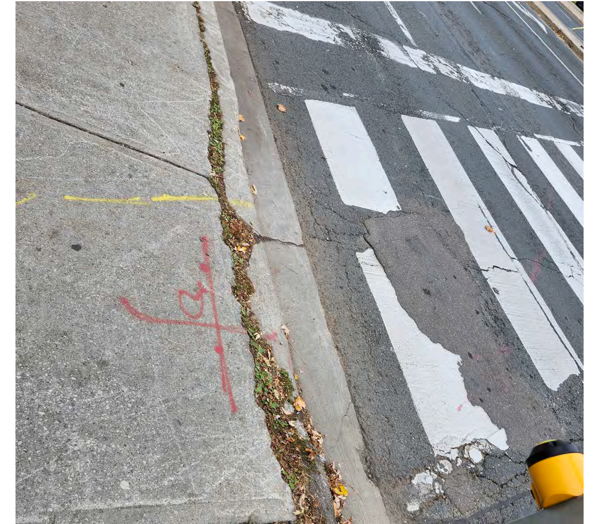
Improper Curb Depression
