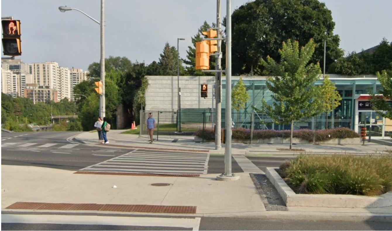
Future LRT entrance, north east corner of Eglinton / Allen
