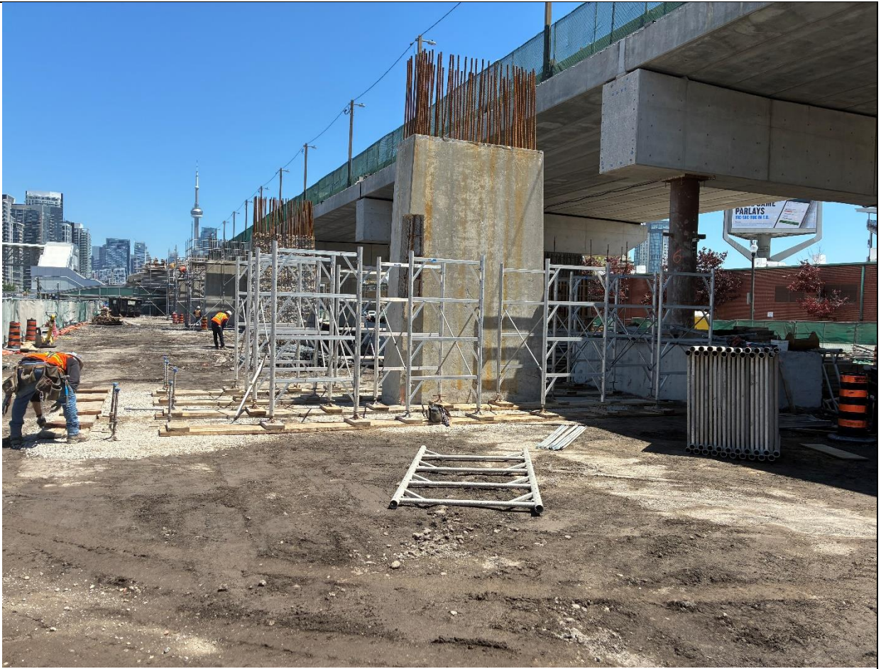
Stage 3 Scaffolding installation for bent cap construction
