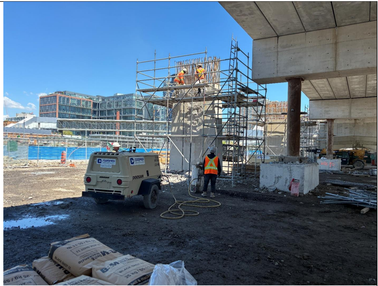
Stage 3 Bent cap concrete removals
