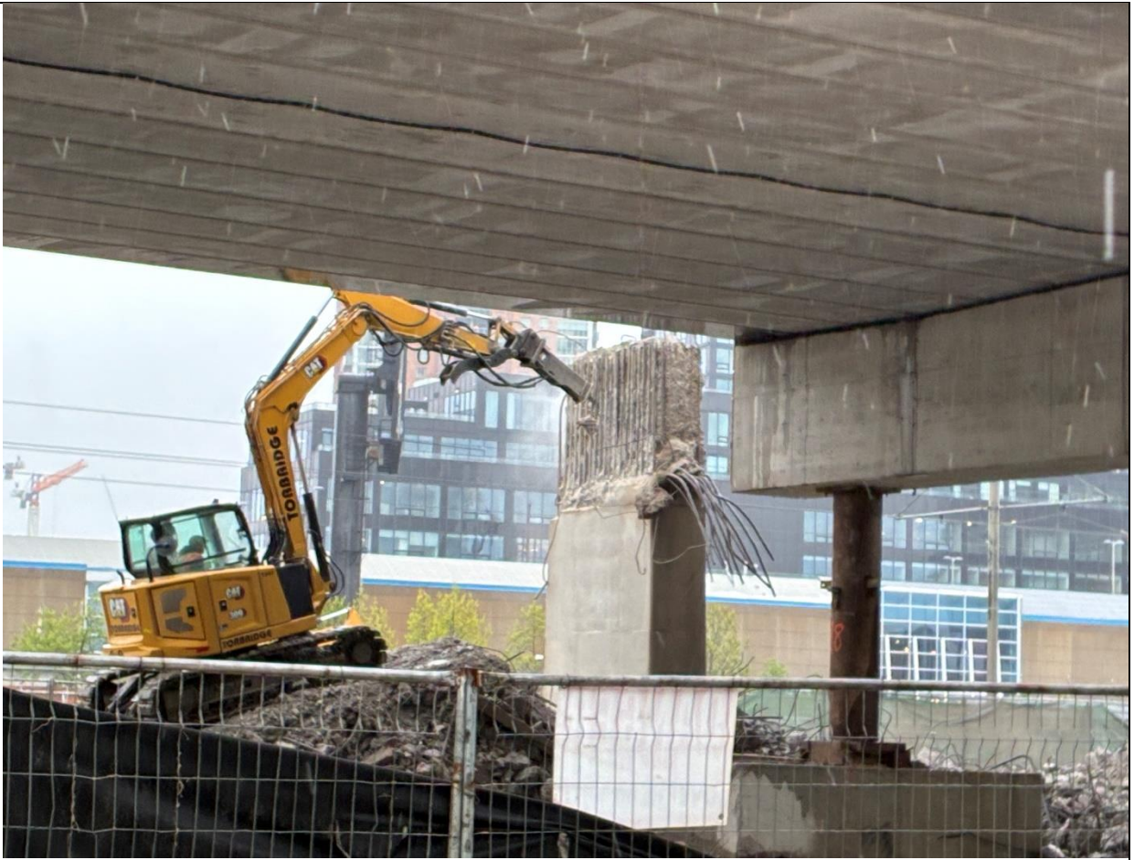
Stage 3 Bent cap demolition
