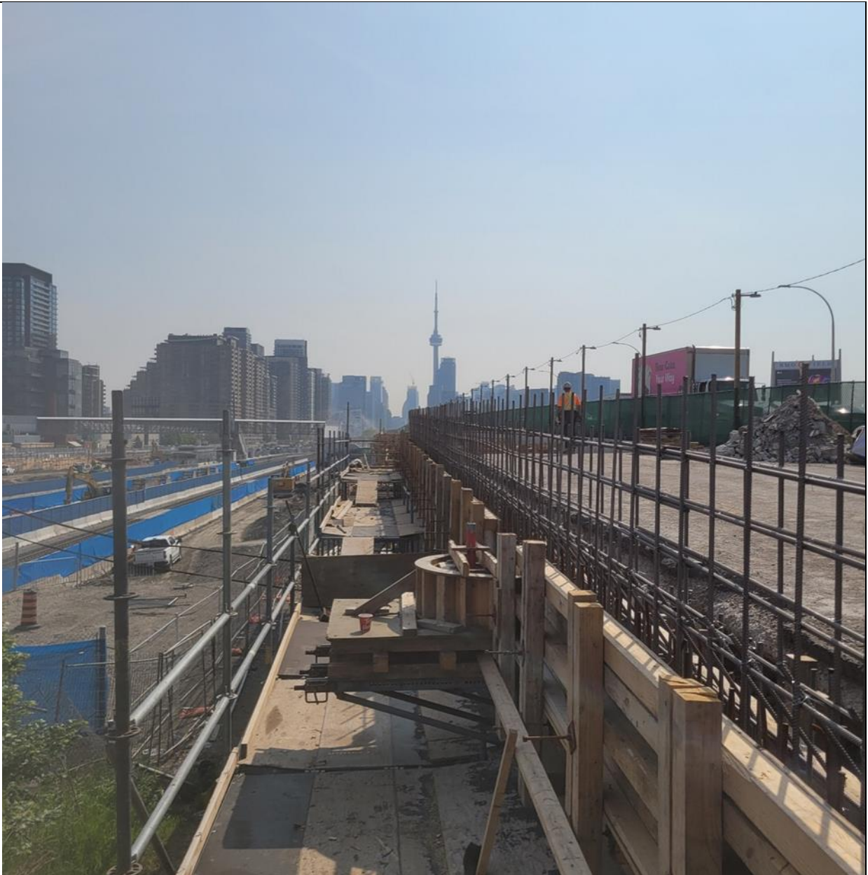
Stage 3 bent cap scaffolding installation
