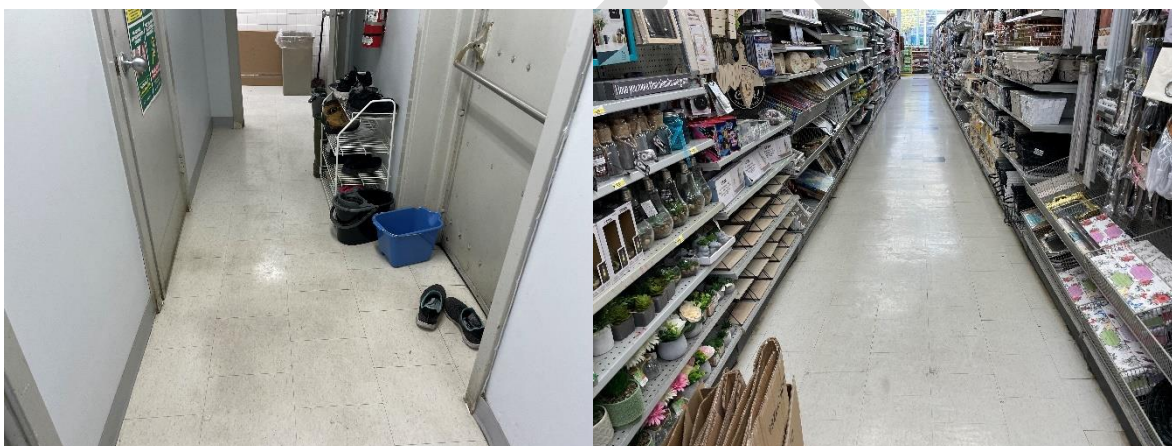
Photograph No. 2.1 and 2.2: View of asbestos-containing Off-white colour vinyl floor tiles identified throughout the mezzanine level and ground floor of the subject building.
