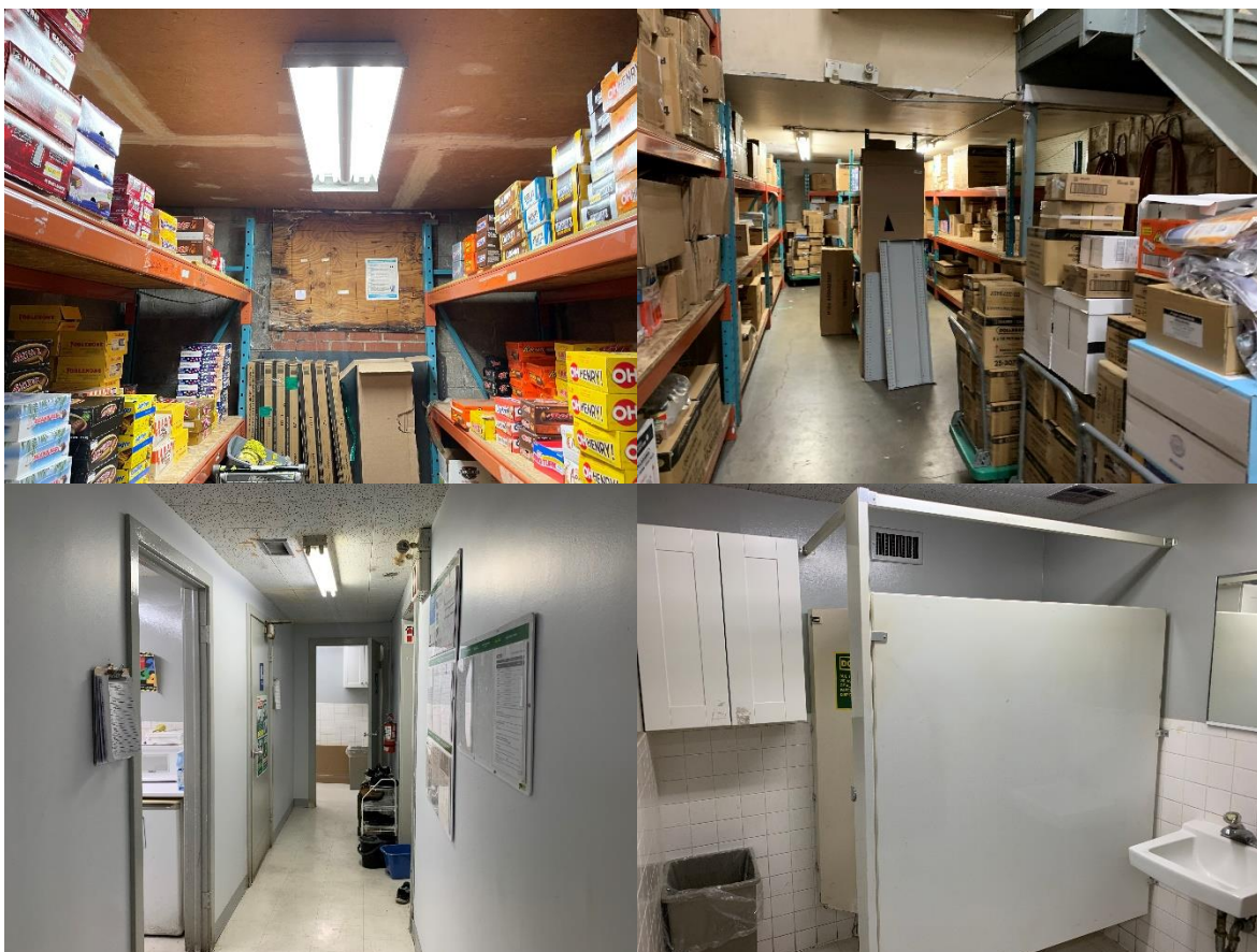
Photograph No. 4.1, 4.2, 4.3 and 4.4: View of asbestos-containing drywall/gypsum wallboard and ceiling board identified throughout mezzanine level and ground floor of the subject building.
