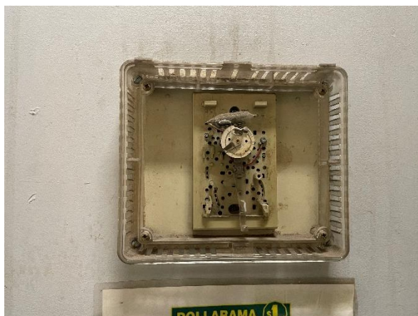
Photograph No. 6: View of a thermostat switch containing a single vial of liquid mercury.
