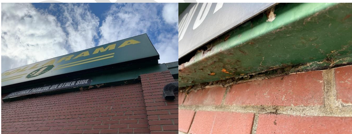
Photograph No. 5.1 and 5.2: View of asbestos-containing white caulking associated with Dollarama signs was identified on the exterior of the subject building.
