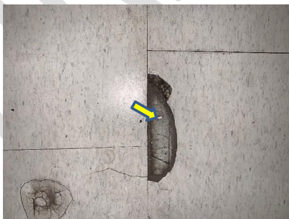
Photograph No. 3: View of asbestos-containing white vinyl floor tiles (2 nd layer) identified underneath off-white asbestos containing vinyl floor tiles throughout the retail area on the ground floor of the subject building.
