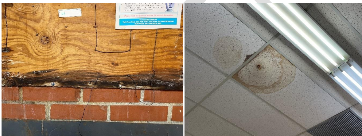
Photograph No. 7.1 and 7.2: Visible mould Growth and signs of water damage observed on the building materials within the subject building.
