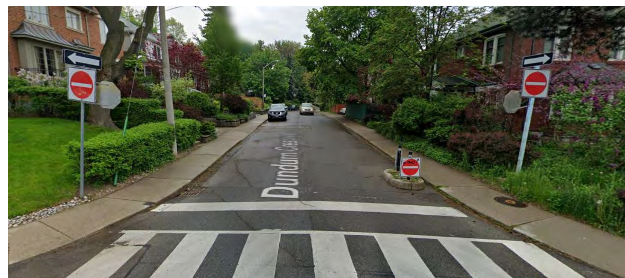
Curb extension to reinforce a directional closure
