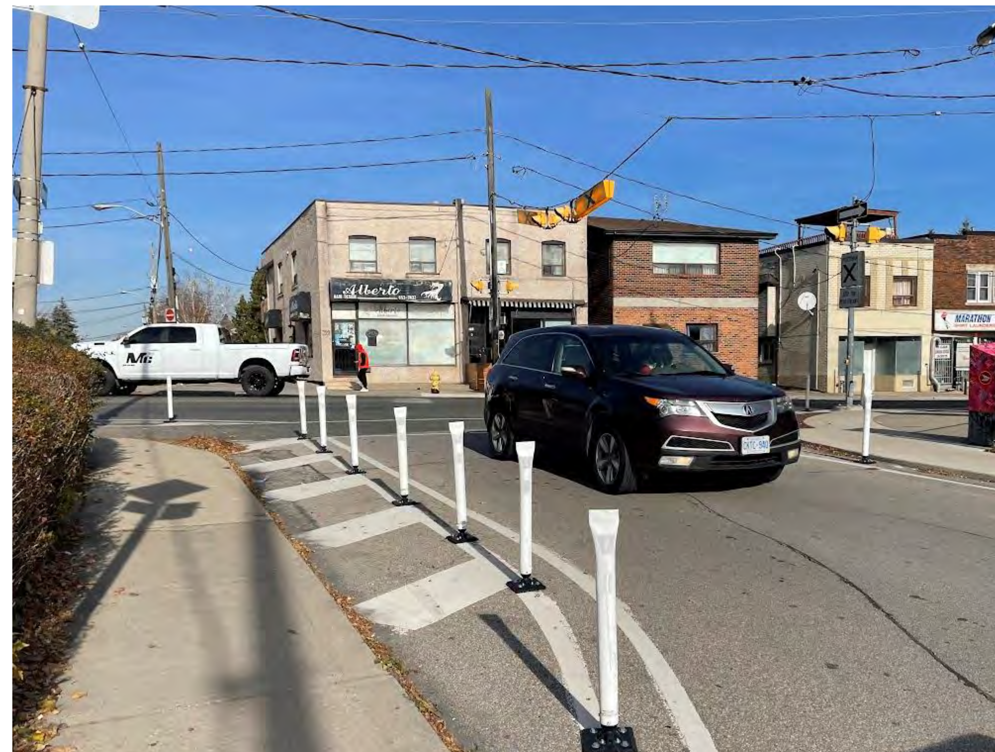
Curb extension with quick-build materials
