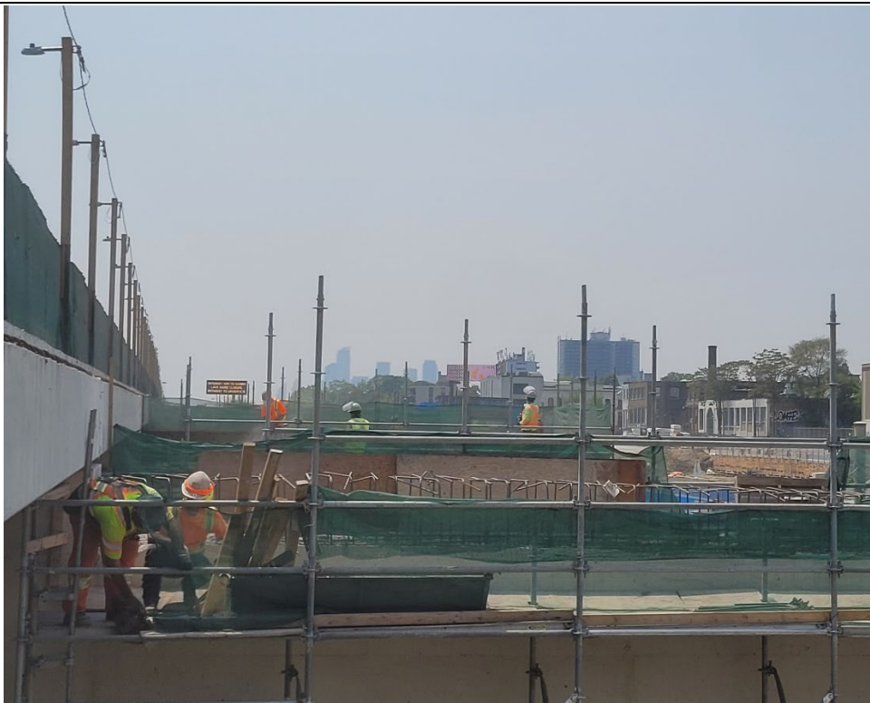
Stage 3 Workers are installing steel dowels—short reinforcing bars—into the top of a concrete bent. These dowels will help connect the new concrete cap to the existing structure, making it stronger and more stable
