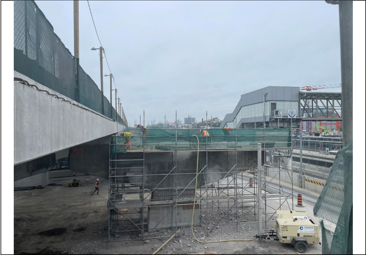
Stage 3 Bent 16 more top of bent cap concrete removals
