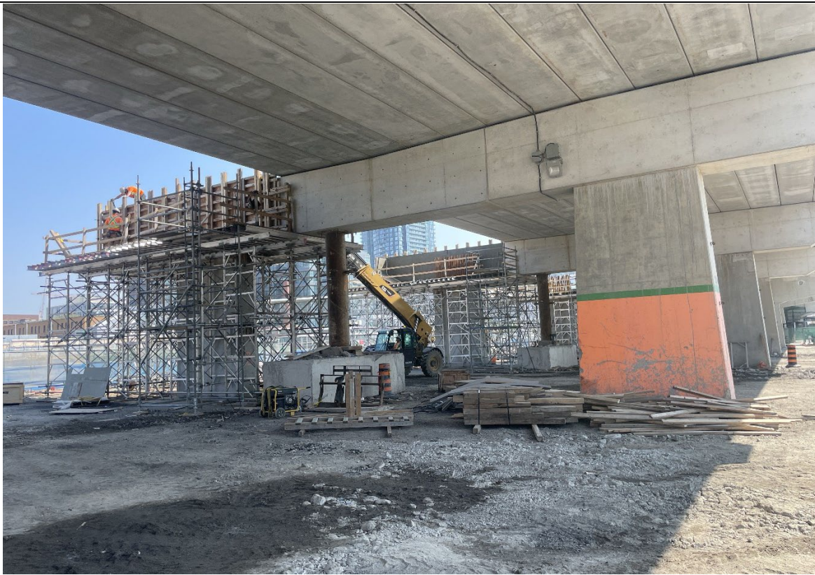
Stage 3 Wooden panels (formwork) that were used to hold poured concrete in place are now being removed. This happens once the concrete has cured (hardened) and is strong enough to support itself. Removing the forms reveals the newly built concrete structure.
