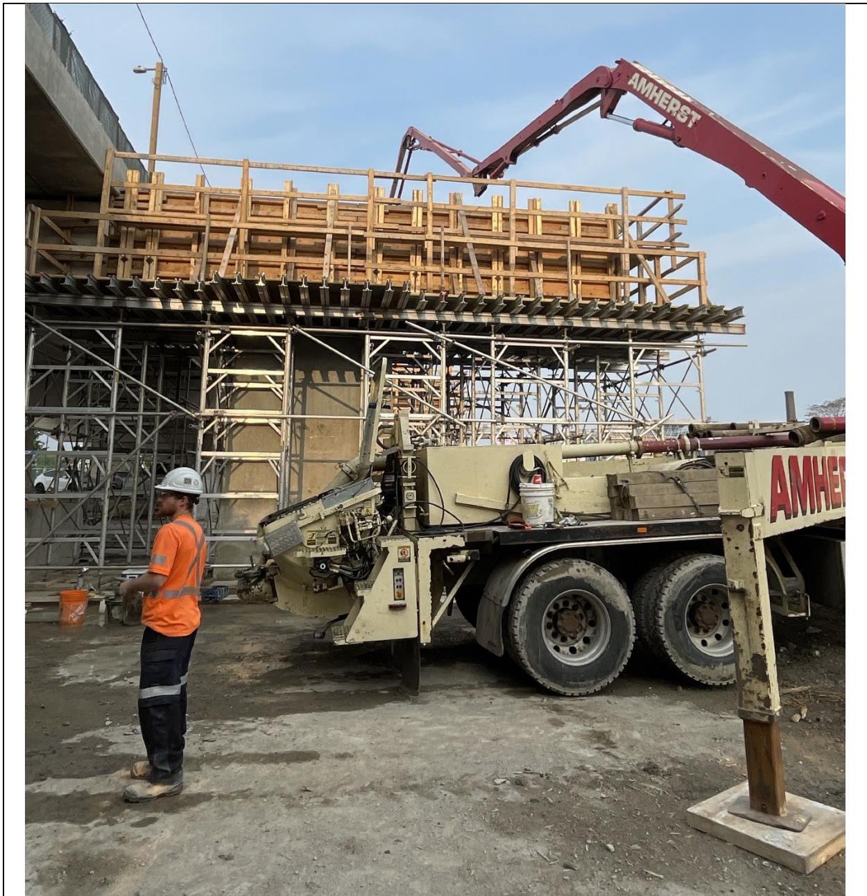
Stage 3 New concrete is being poured into the prepared area to form a new bent cap
