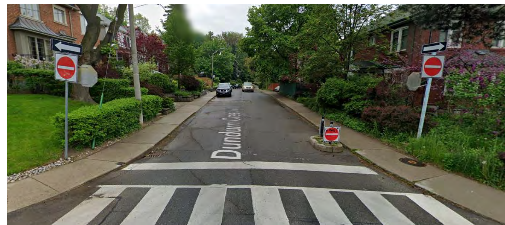
Curb extension to reinforce a directional closure
