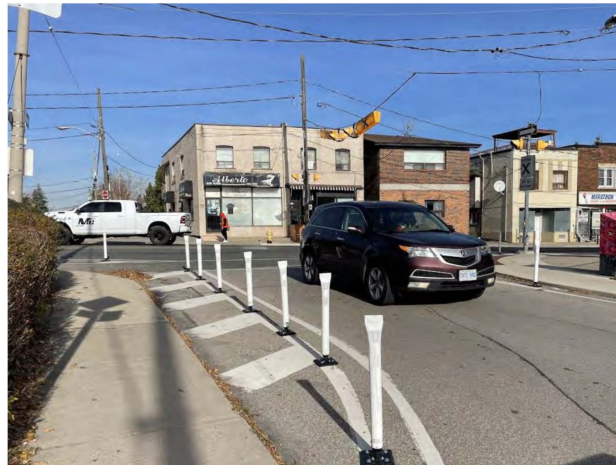
Curb extension with quick-build materials
