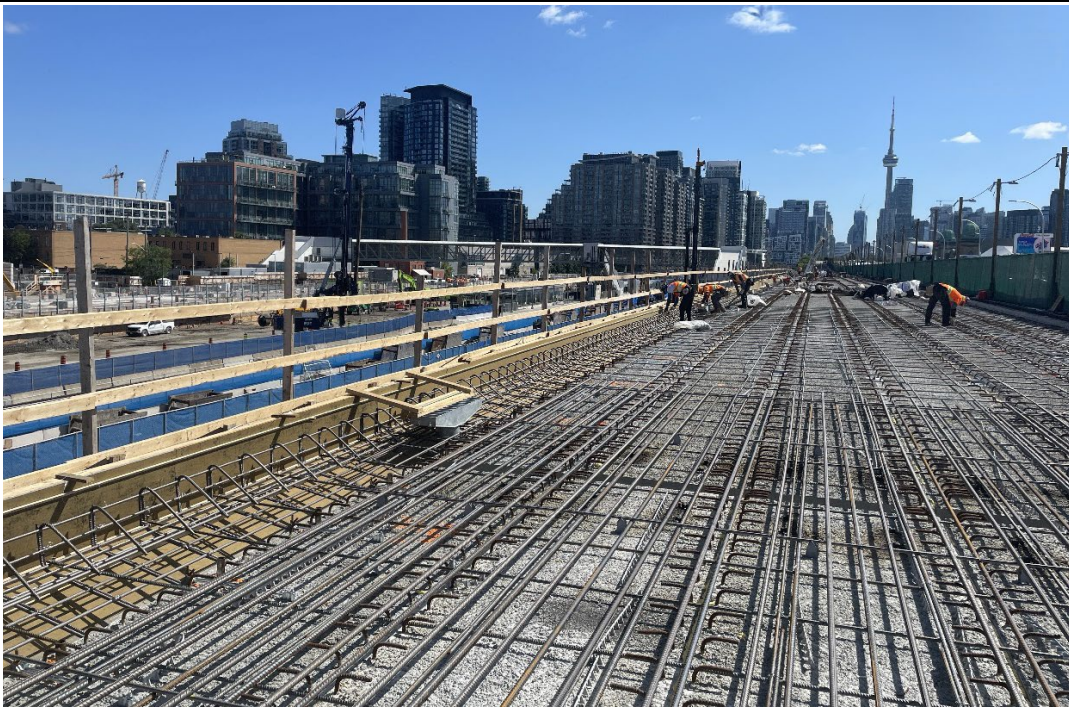
Stage 3 Bridge Deck Reinforcement Installation
