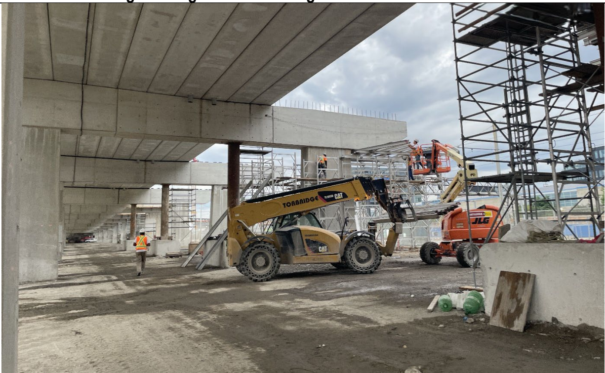
Stage 3 Bent Cap Falsework Removal
