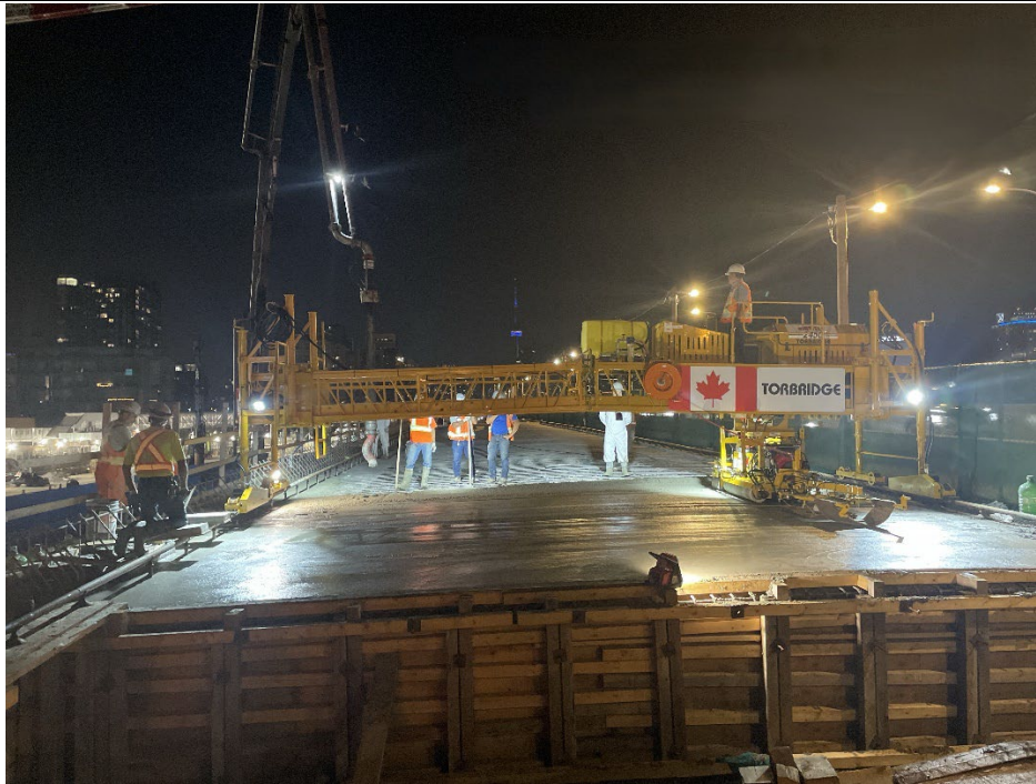
Stage 3 Bridge Deck Concrete Placement
