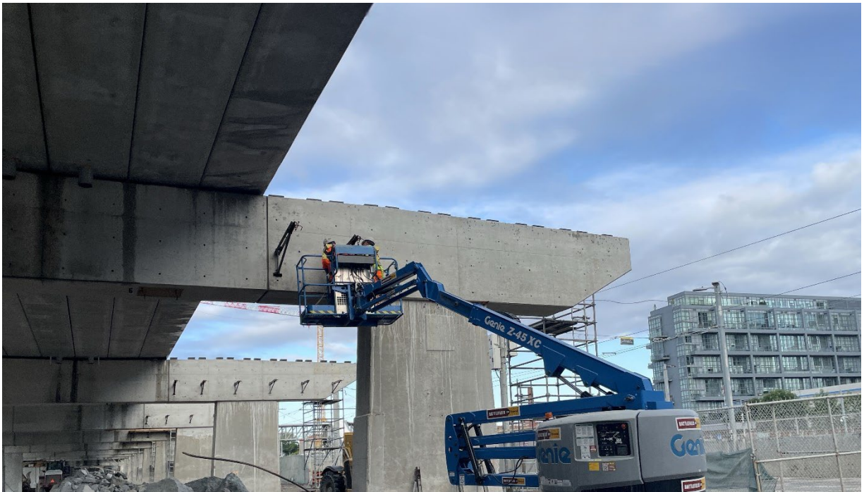
Stage 3 Removal of access platform brackets
