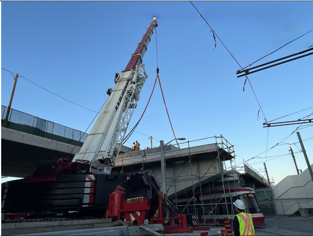
Stage 3 Girder Erection
