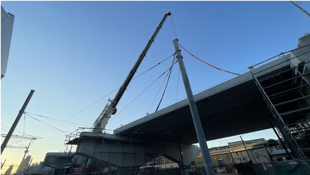
Stage 3 Girder Erection
