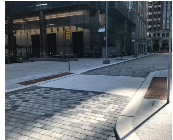
Figure 3.31 Raised Crosswalk, Temperance St, Toronto, ON
