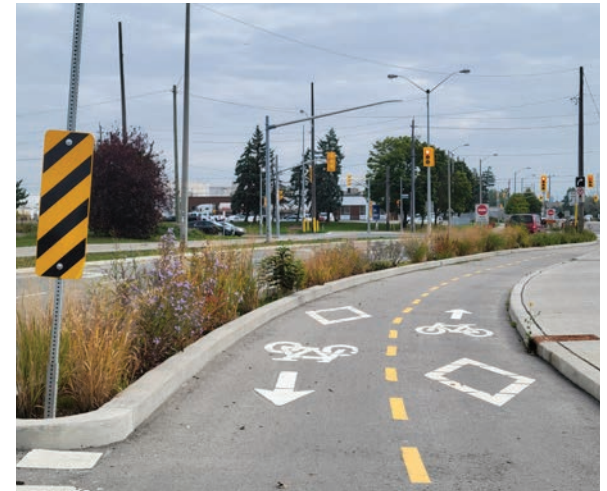
Figure 3.25 Green Gutter and Bikeway, Toronto, ON
