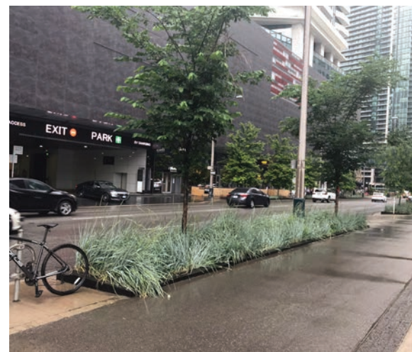
Figure 3.23 Tree Planter with Curb Openings to Allow for Rainwater Collection, Toronto, ON
