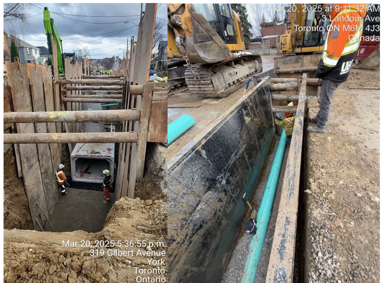
Left: Installation of local storm sewers (March 2025)
