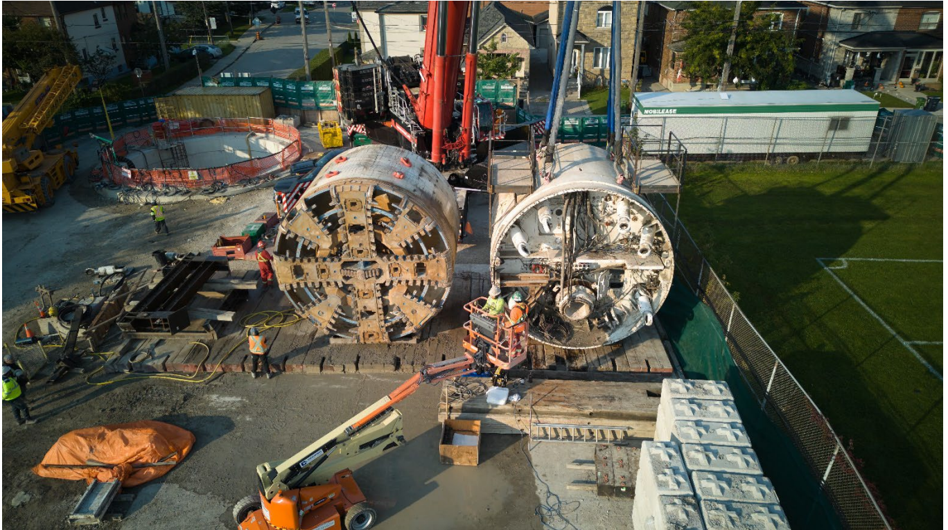
Tunnel Boring Machine after being extracted from the Bicknell Avenue and Nashville Avenue Shaft upon completion of tunneling (October 2024)
