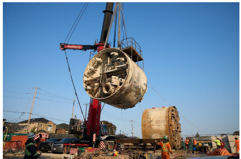
Extraction of the TBM from the Bicknell Avenue and Nashville Avenue shaft (October 2024)
