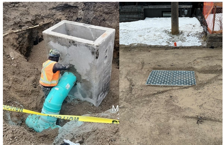
Left: Installation of High Capacity catch basin at Glenholme Avenue (March 2025)
