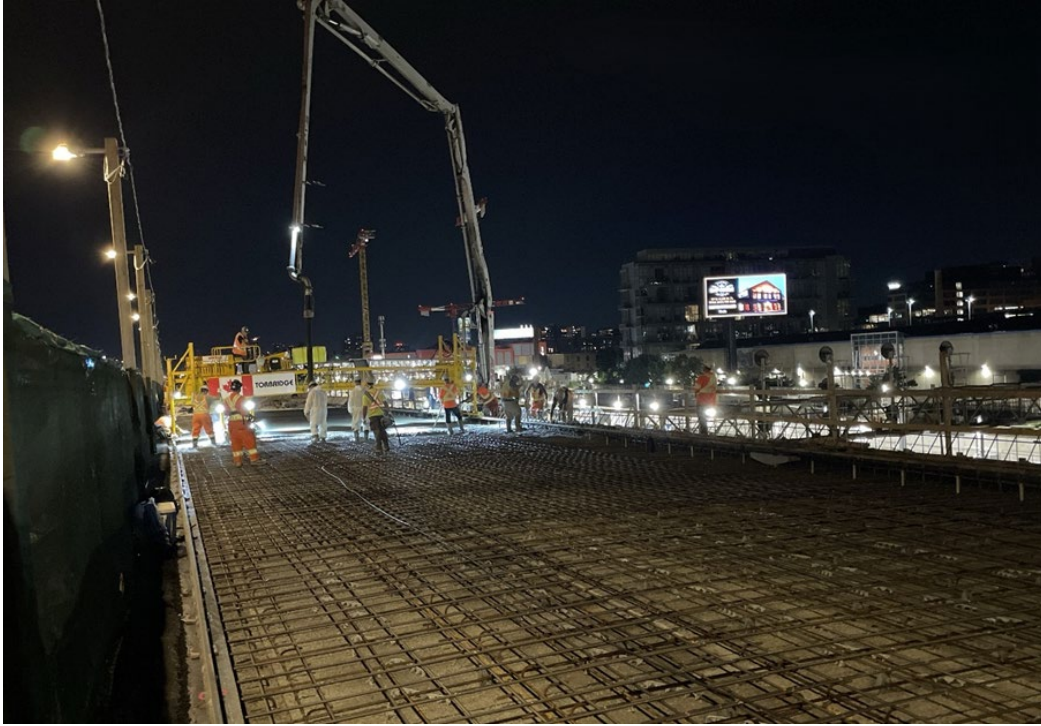
Stage 3 Bridge Deck Concrete Placement
