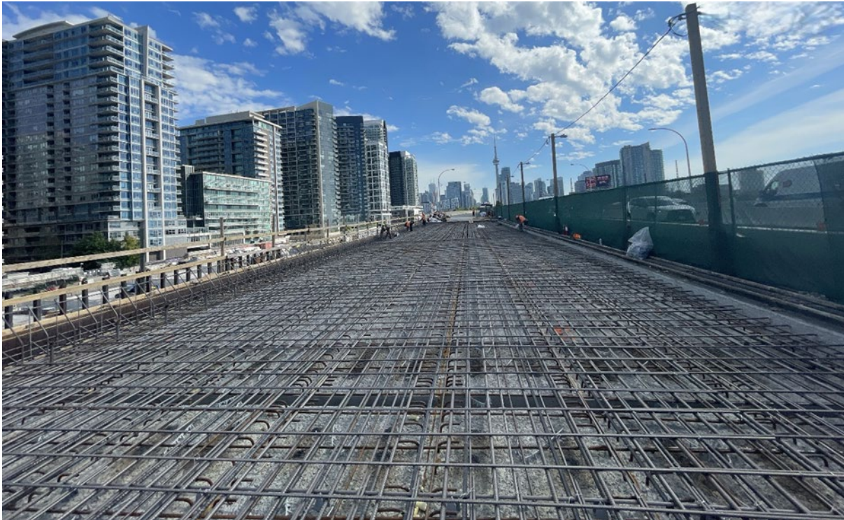
Stage 3 Bridge Deck Reinforcement Installation
