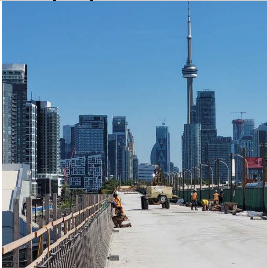
Stage 3 barrier wall reinforcement installation
