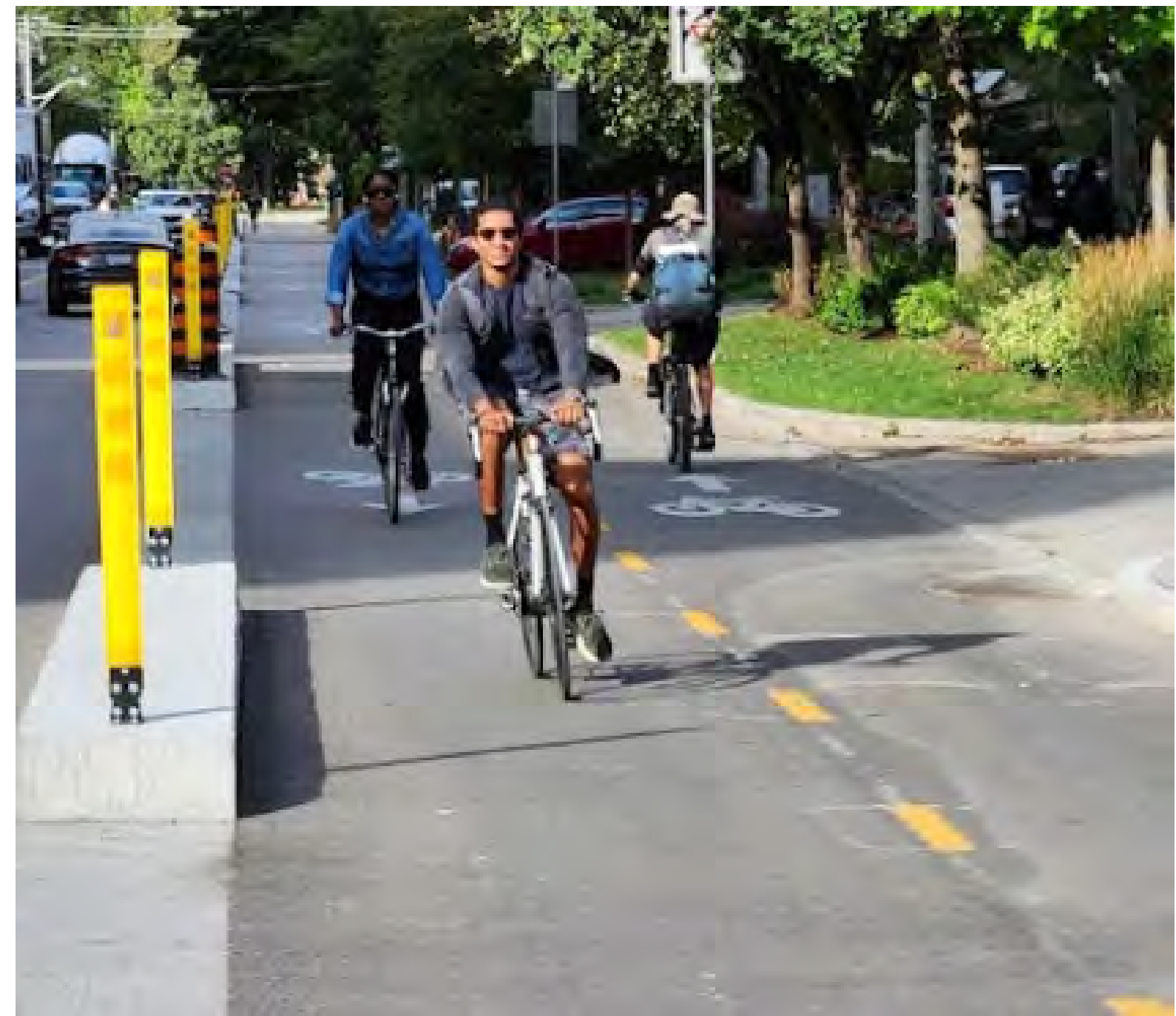
Concrete Separation Example
