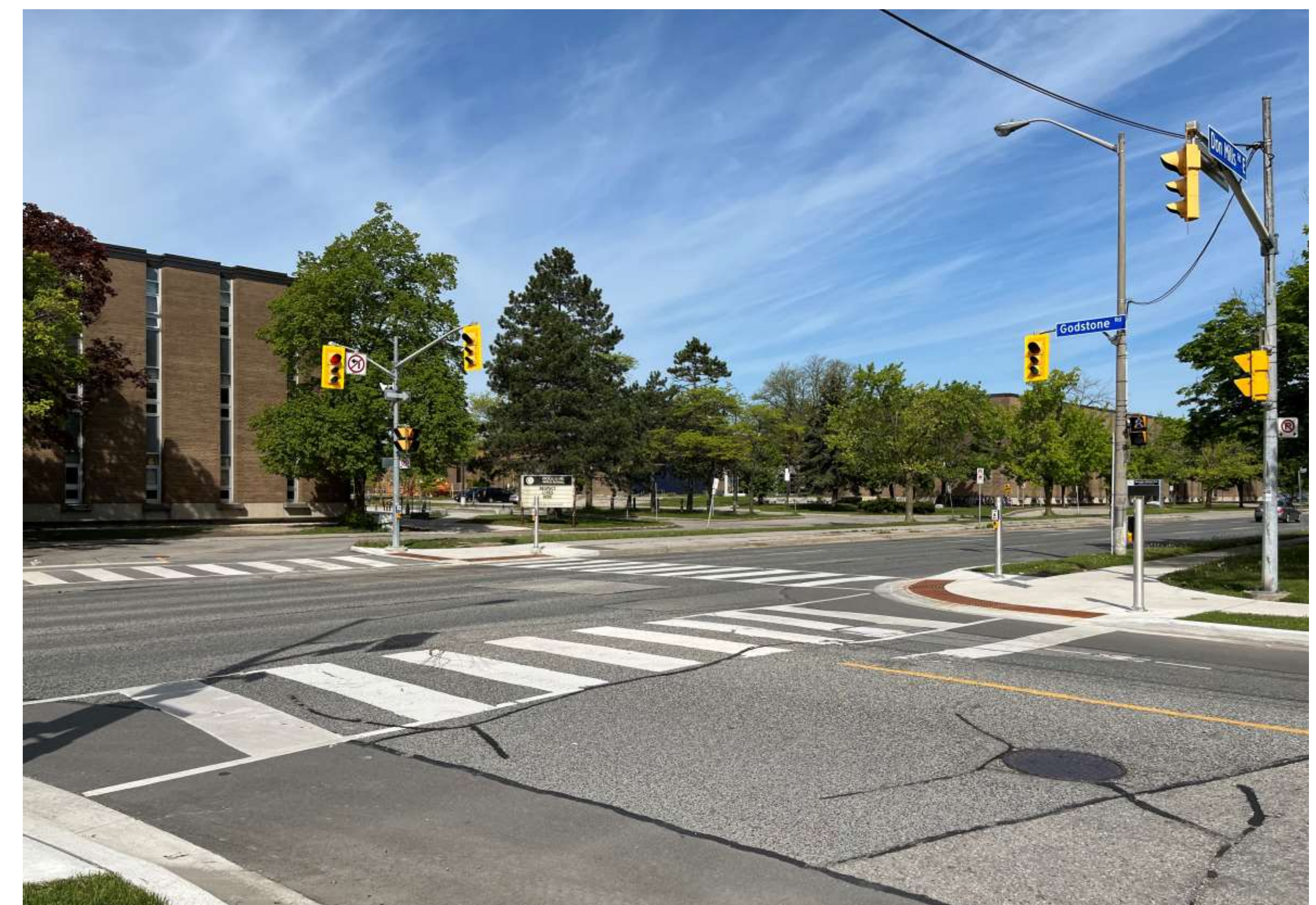
Signalized Intersection at Don Mills Road & Godstone Road
