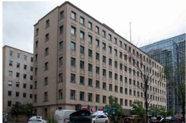
The Crown Life Building at 120 Bloor St. E. (CBCollective 2021).
