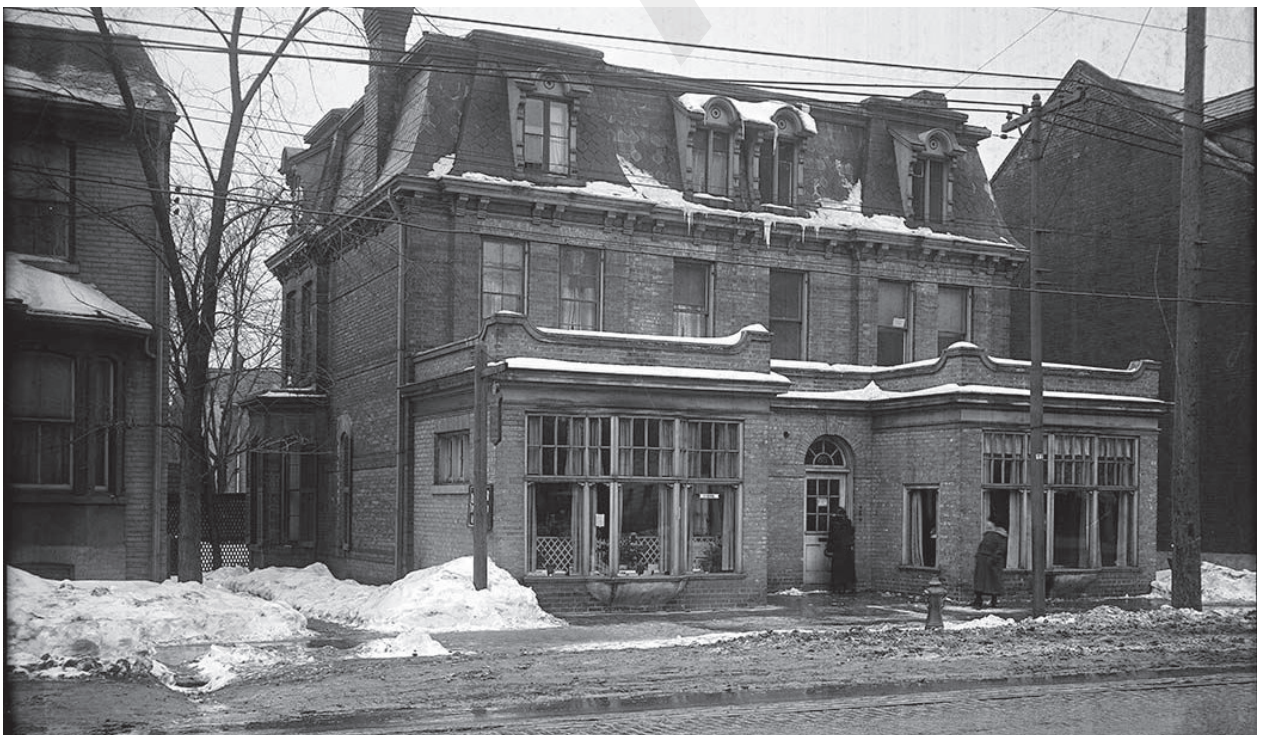
Figure 31: 1924 photograph of 83-85 Bloor Street West, an example of a former residence using a commercial addition to support new uses ( City of Toronto Archives ).
