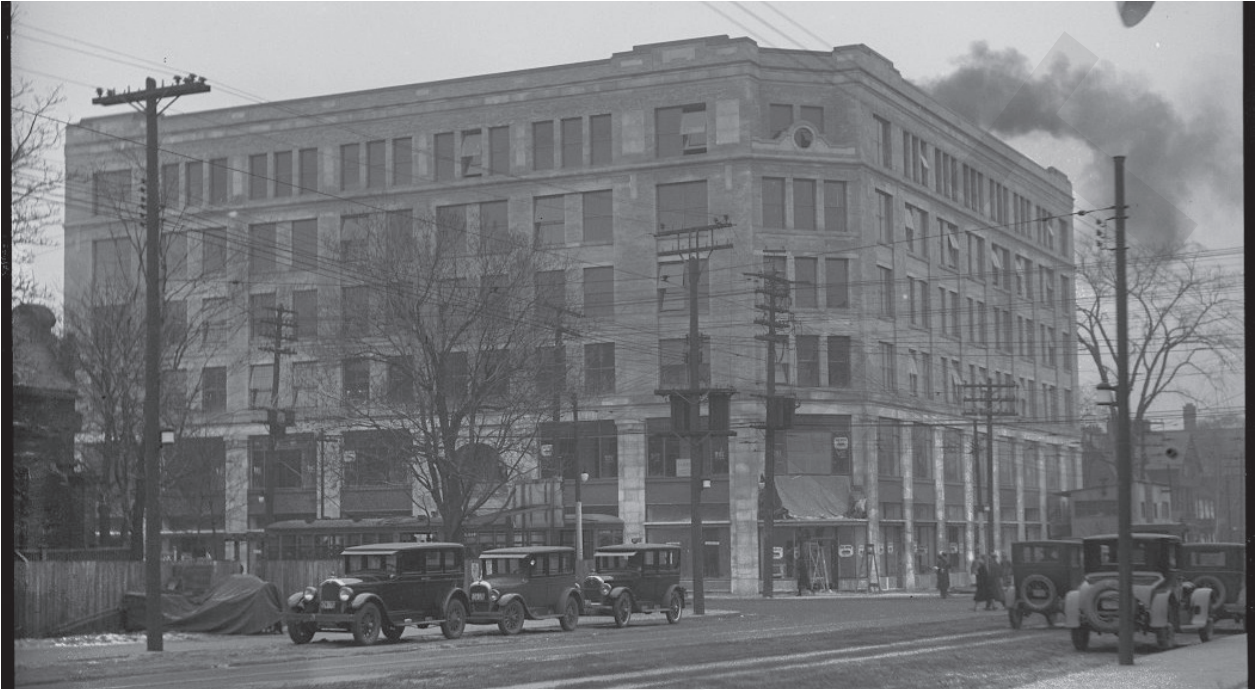
Figure 34: 1926 photograph of the 6-storey Bloor Building still under construction at the southeast corner of Bay and Bloor streets ( City of Toronto Archives ).
