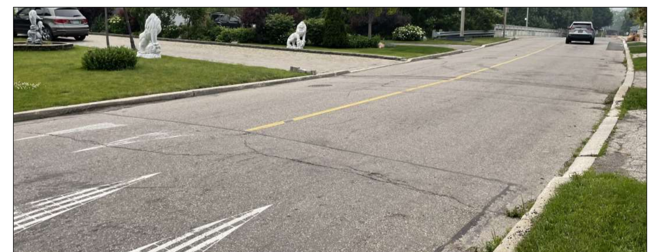
Speed humps on Queens Drive
