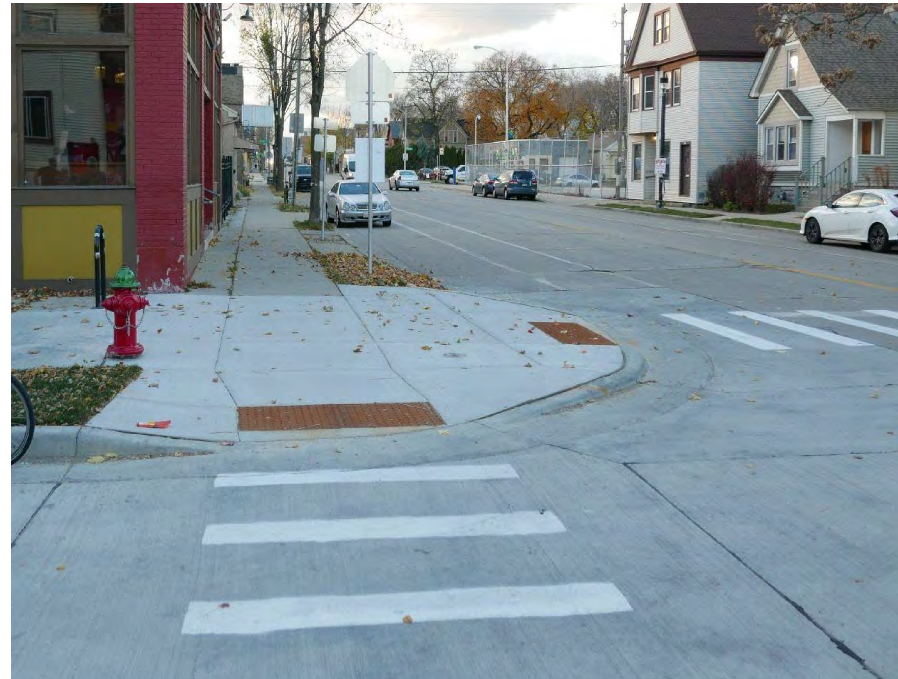
An example of a curb extension at an intersection
