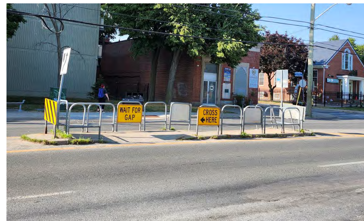
Pedestrian refuge island on Danforth and Robinson Avenue
