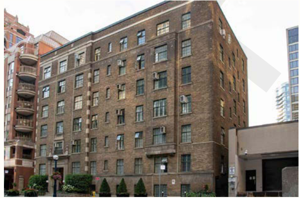
Apartment building at 2 Sultan St. (CBCollective 2021).
