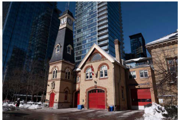
The Yorkville Fire Hall at 34 Yorkville Ave. (CBCollective 2022).
