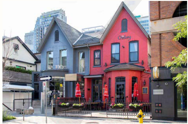
Former residential semi-detached at 117-119 Yorkville Ave. (CBCollective 2021).
