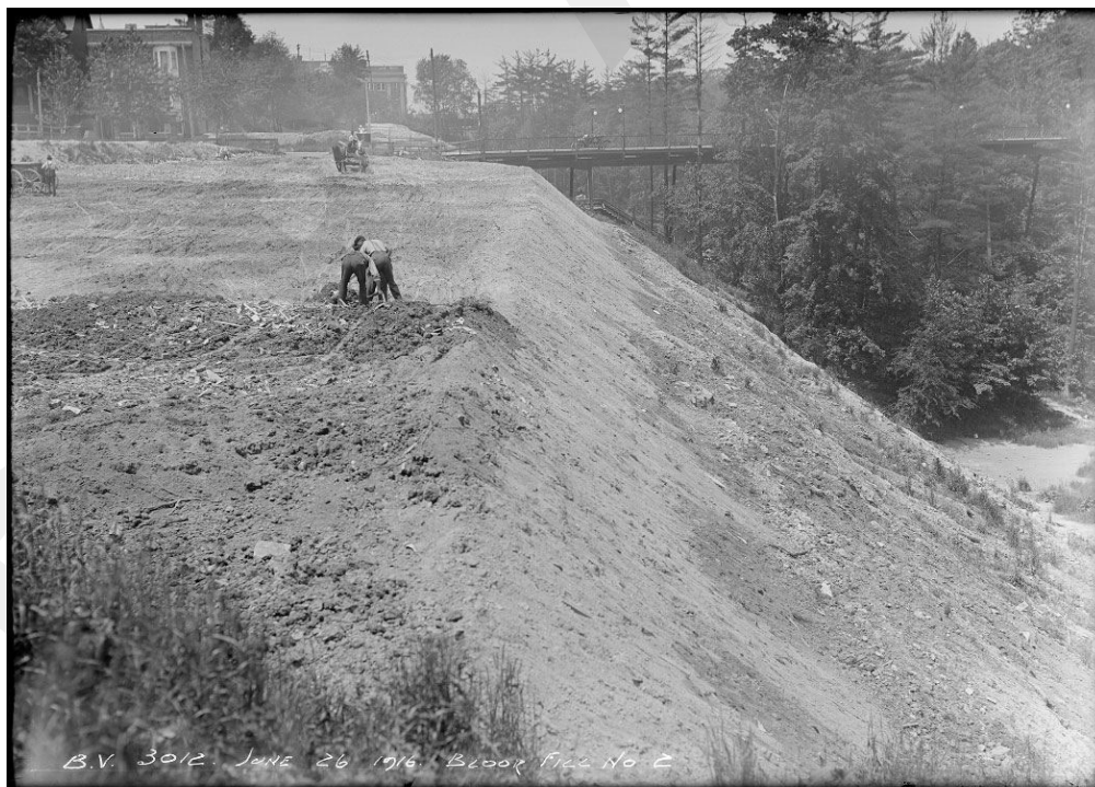
Figure 23: 1915 archival photograph looking northeast to Bloor and Sherbourne streets, with the Toronto Dominion Bank building in the background. In the foreground an embankment is being build-out over the Rosedale Ravine to support the extension of Bloor Street East ( City of Toronto Archives ).
