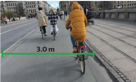
Figure 2.3 ABOVE: Lower limit width of raised cycle track. People cycling cannot ride side by side and stronger riders cannot pass. Figure 2.4 BELOW: Upper limit width of raised cycle track. Here, riders can be side by side and pass. While both facilities provide sufficient protection, the second is more comfortable.
