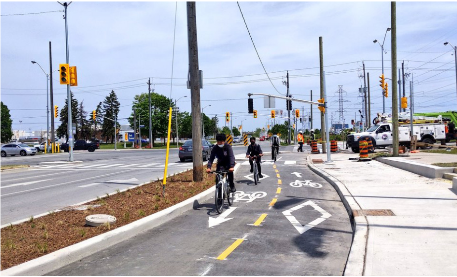
Figure 2.8 Along the Finch Hydro Corridor, another Major City-Wide Cycling Route, a new direct and intuitive cycle track and wider sidewalks were built. Careful attention was paid to separate pedestrians and people cycling, as the volumes of both are anticipated to grow overtime.
