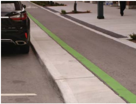
Figure 3.13 A sidewalk elevation cycle track with a concrete buffer adjacent to parking.
