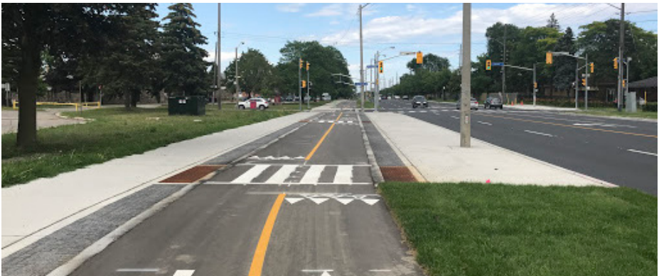
Figure 3.23 A multi-use path adjacent to a sidewalk with tactile unit paver as separation.
