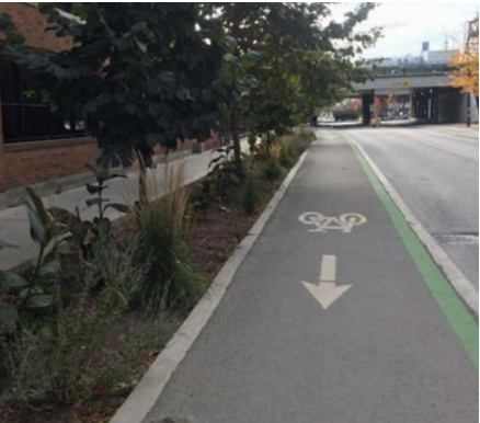
Figure 3.9 A sidewalk elevation cycle track separated by a planting strip.
