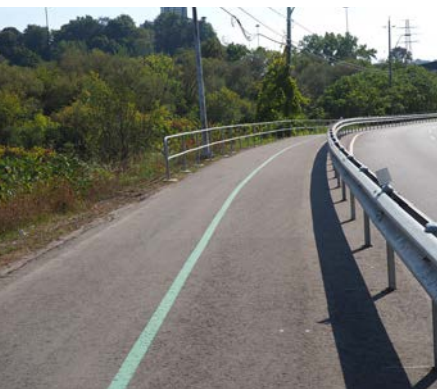
Figure 3.22 A multi-use path separated with a guard rail.
