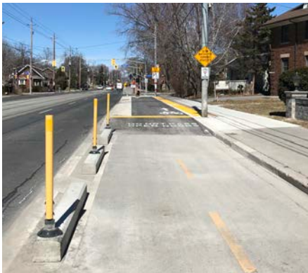
Figure 3.20 A precast barrier curb and flex bollards separation treatment.
