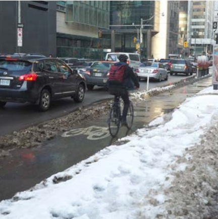
Figure 3.26 A cycle track with snow stored on both sides of the facility.
