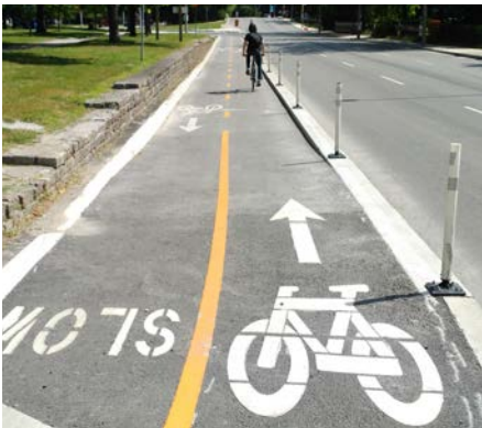
Figure 3.18 A poured barrier curb and flex bollards separation treatment.
