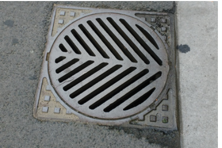
Figure 3.55 A catch basin with herring bone grates.
