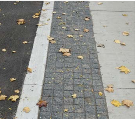
Figure 3.8 A band of visually contrasting, cane detectable unit pavers adjacent to a sidewalk elevation cycle track.
