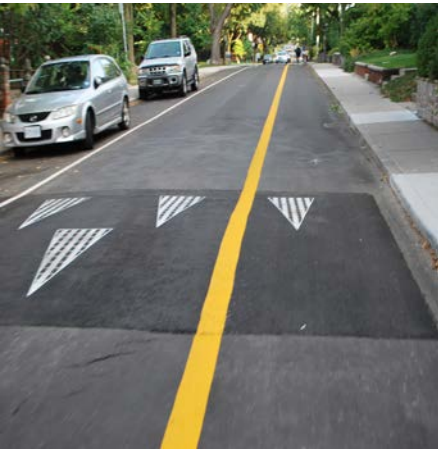
Figure 3.48 A contra-flow bicycle lane along with additional traffic calming.
