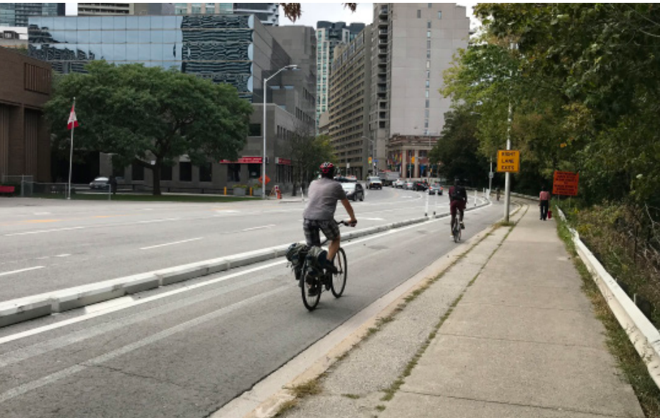
Figure 2.7 Bloor Street, Danforth Avenue and Kingston Road form an east-west Major City-Wide Cycling Route. In 2021, the existing Bloor Street East bike lanes were widened to 2.1 -2.4 metres and protection was added to align with Ontario's best practices and the City's On-Street Bikeway Guidelines.
