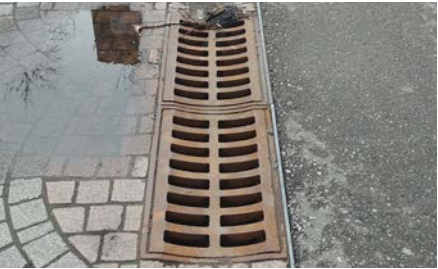
Figure 3.7 A narrow catch basin adjacent to a bi-directional cycle track.
