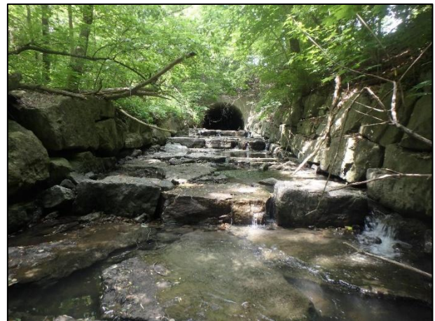
Figure 4-50: Armourstone Bed works over the 675 mm Sanitary Sewer Crossing, Constructed as a Series of Cascades
