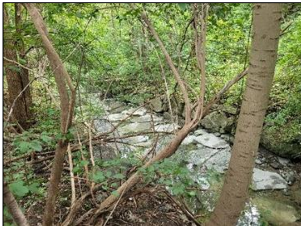
Figure 4-51: Degraded Armourstone Bed and Bank Treatments
