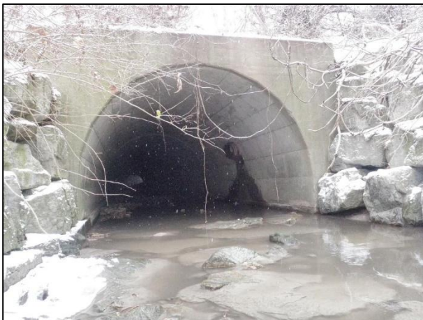
Figure 4-49: Arched Culvert conveying Flows under the Intersection of Bayview Avenue and Finch Avenue
