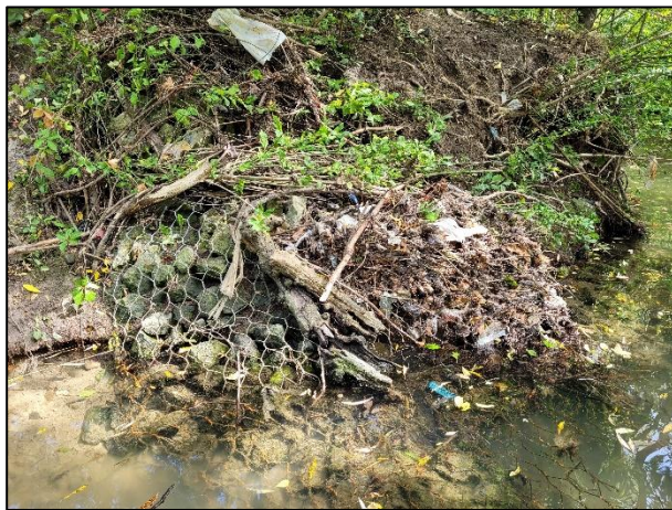
Figure 4-55: Failed Gabion Basket Bank Protection
