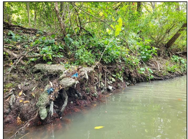
Figure 4-58: Undermined and Emptied Gabion Baskets Upstream of Watermain Crossing
