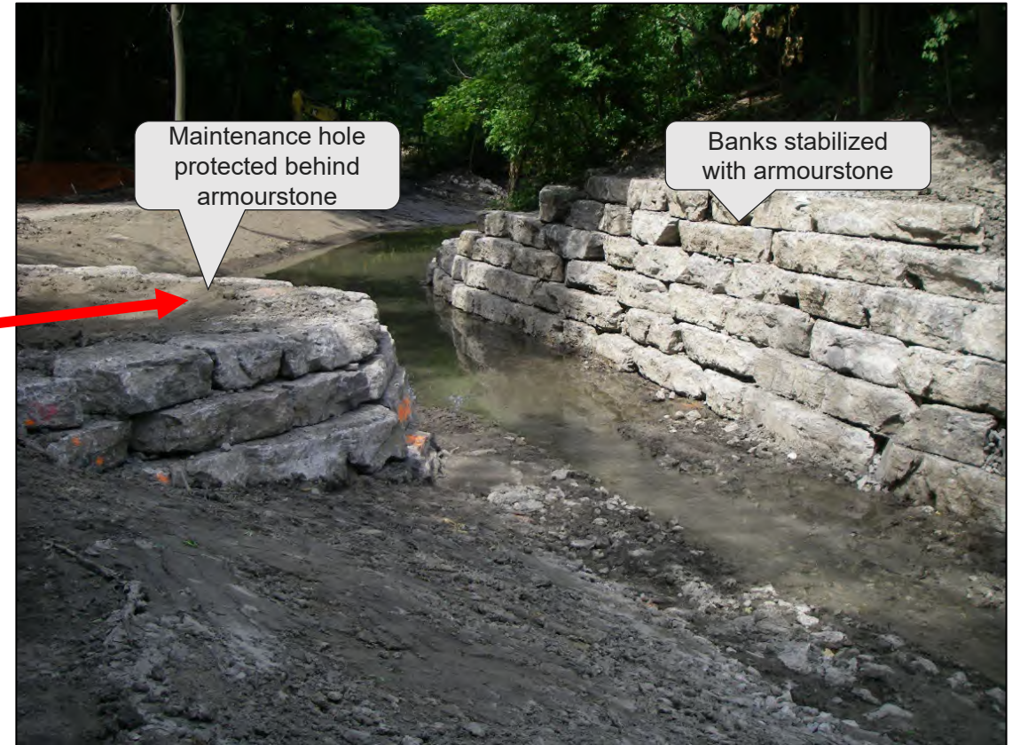
Massey Creek – Creek has been realigned away from maintenance hole with Armourstone walls built as bank protection (post-construction but pre-restoration)
