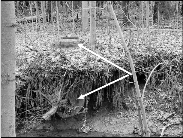
Exposed manhole in the bank
