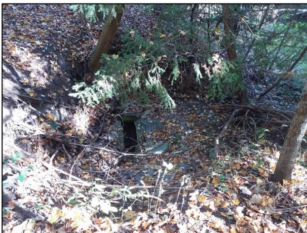
Figure 4-15: Location of Visible Pipe Detachment Upslope of the Outlet
