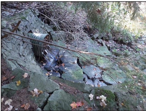
Figure 4-13: Stormwater Outlet Clogged with Organic Debris
