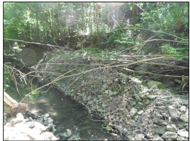
Figure 4-8: Undercut Gabion Basket Retaining Walls Slumping Downwards into Channel
