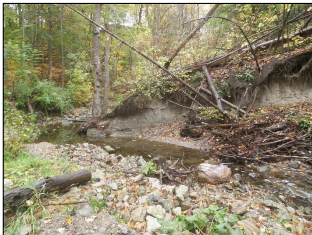
Figure 4-3: Significant Bank Erosion Between the Exposed Sewer Crossing and Downstream Maintenance Hole
