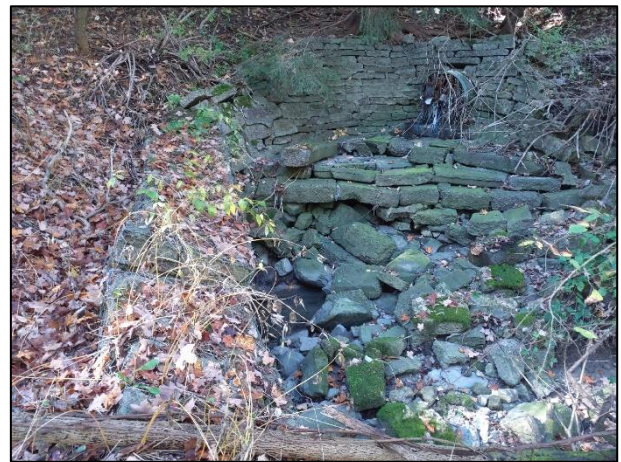
Figure 4-14: Degraded Outfall Channel with Loose Angular Stone
