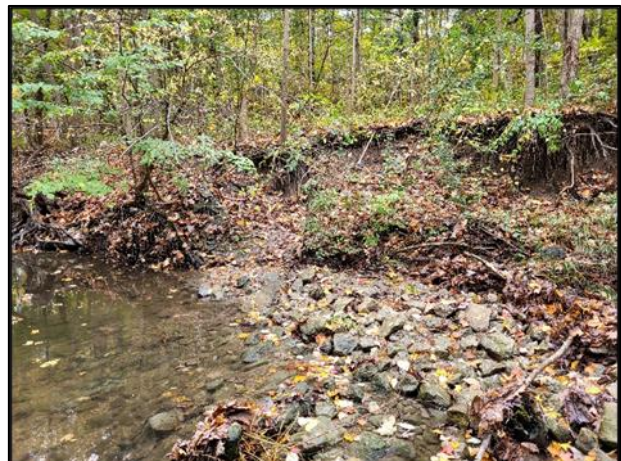
Figure 4-10: Failed Gabion Basket Retaining Wall and Widened Channel due to Unprotected Eroding Banks Downstream of the Exposed Sewer Crossing
