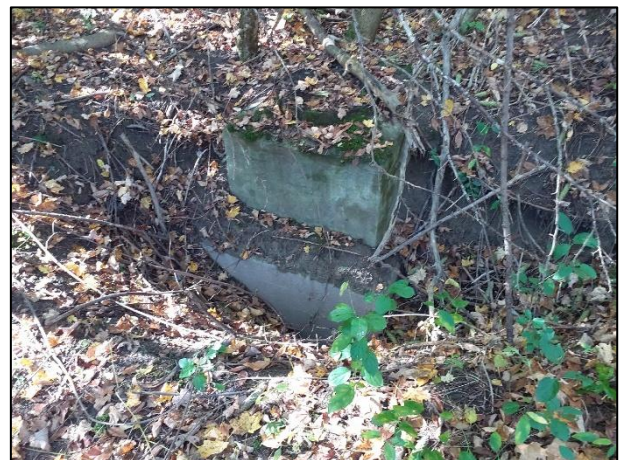
Figure 4-16: Exposed Maintenance Hole in the Slope of Forest Grove Drive Road Embankment
