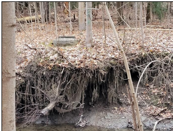
Figure 4-1: Exposed Sanitary Maintenance Hole in Bank
