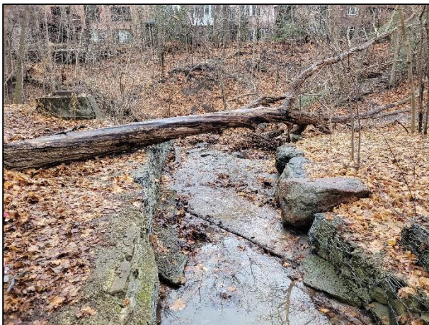
Figure 4-79: Exposure of the Concrete Encasement with Water Flowing into the Crack of the Encasement
