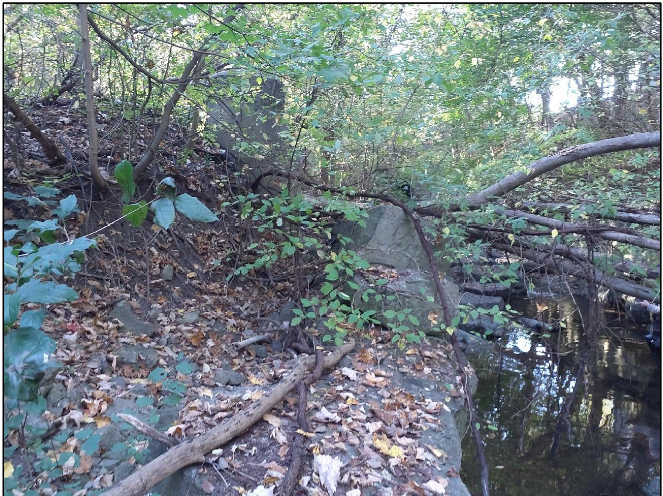
Figure 4-106: Outflanked and Failing Armourstone Retaining Wall Posing Lateral Erosion Risk to 675 mm Diameter Sanitary Sewer, Partial Exposure of Sanitary Sewer Maintenance Hole Present
