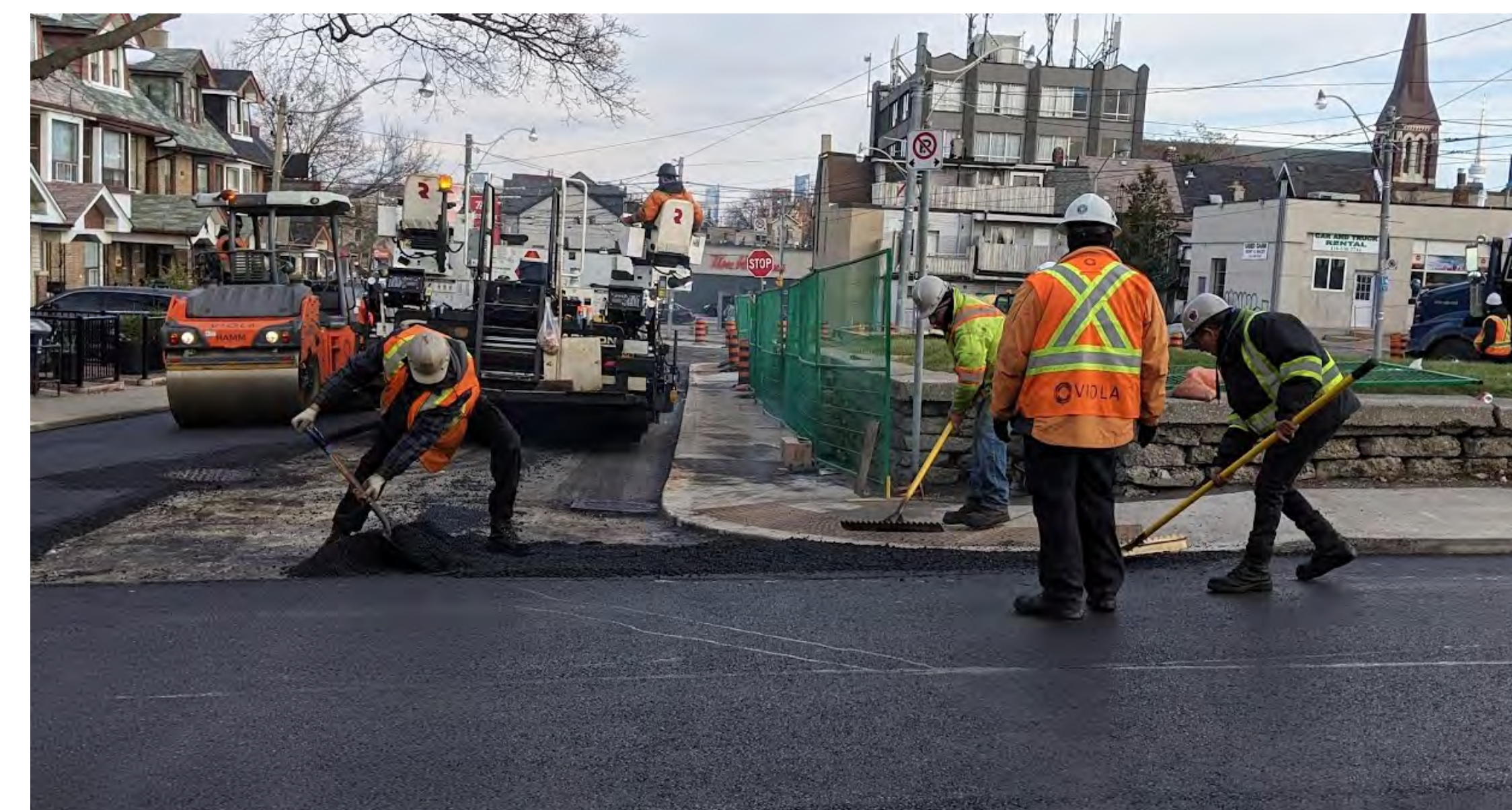
Example of road resurfacing works
