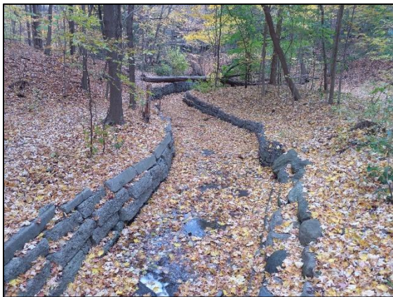
Figure 3-13: Armourstone and Concrete Lined Channel Upstream of the Confluence with Br1
