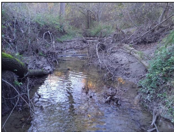
Figure 3-9: Incised Channel Near the Don Confluence Exposing Buried Pipes and Bank Erosion.
