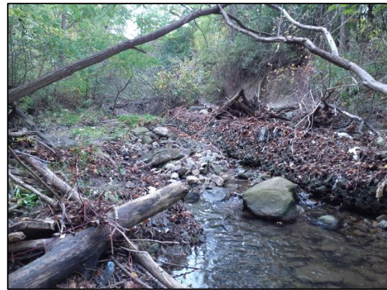
Figure 3-6: Failed Gabion Baskets Through Reach N3
