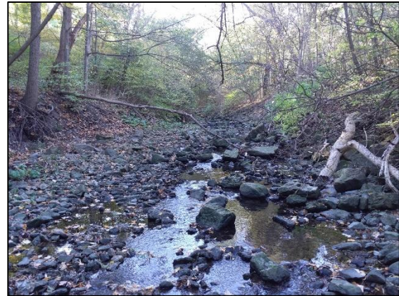
Figure 3-4: Washed-Out Angular Stone and Boulder Treatments in Reach N2
