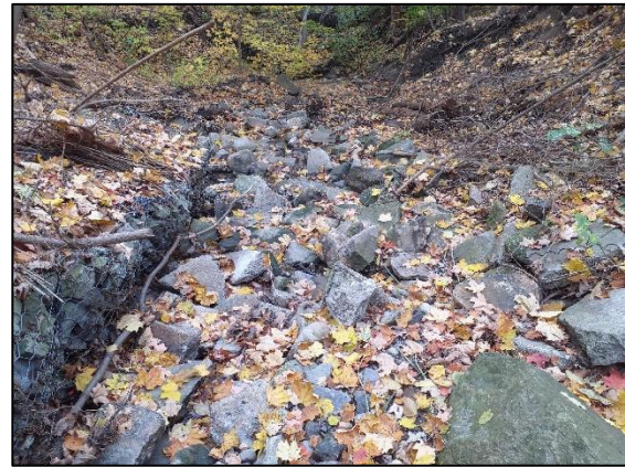
Figure 3-16: Failed Gabion Baskets and Channel Angular Stone in Reach Br4
