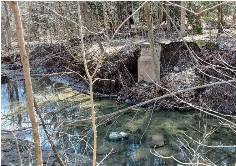
Exposed Maintenance Hole
