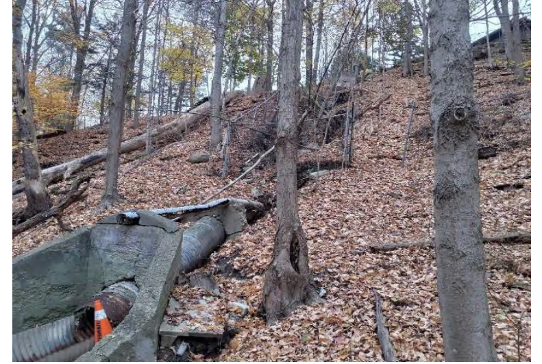
Failing Outfall
