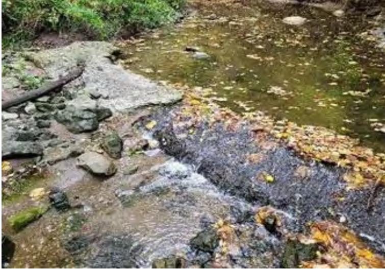
Exposed Sanitary Sewer Crossing
