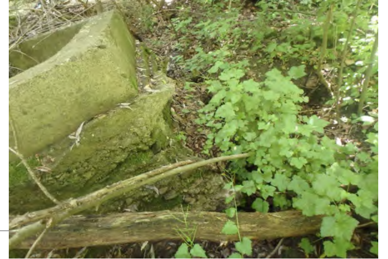
Failed Concrete Outfall Wall
