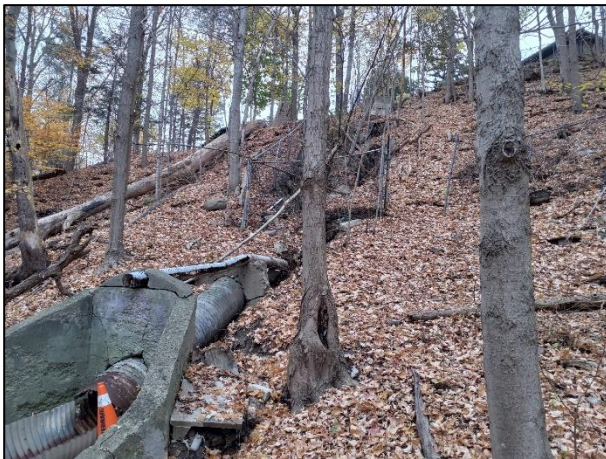
Figure 4-67: Storm Outfall Failure in the Slope of the Valley
