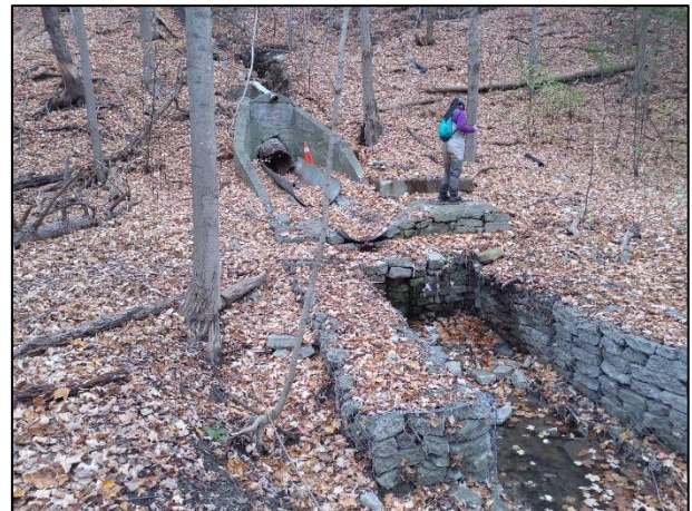
Figure 4-68: Degraded Outfall Channel
