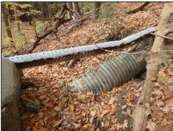
Figure 4-69: Two Failed Pipes Upslope of Headwall
