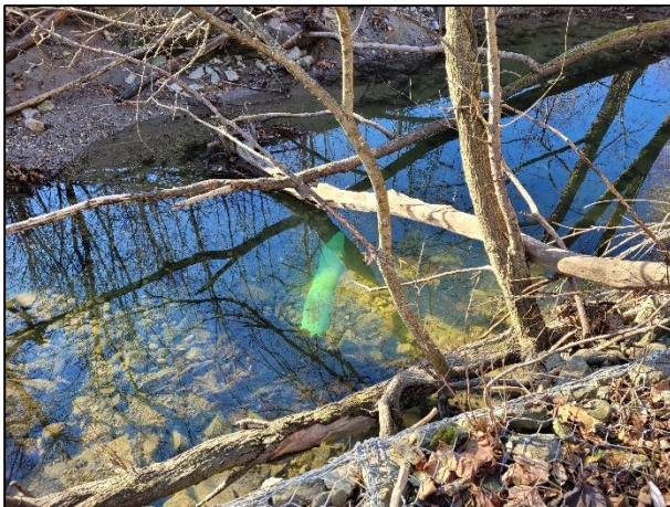
Figure 4-61: Exposed Sewer in Channel Bed Without Visible Encasement
