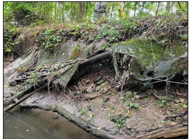
Figure 4-62: Bank Subject to Erosion with Degraded Geotextile Fabric
