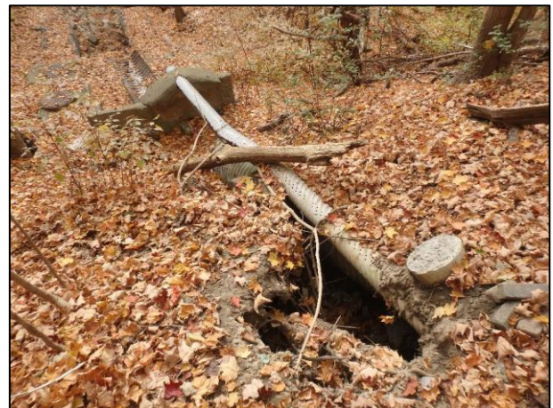
Figure 4-70: Sinkhole Observed Upstream of Headwall Structure
