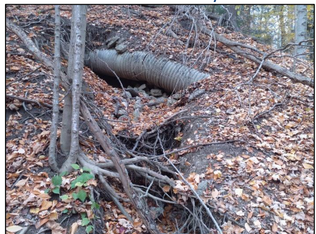
Figure 4-76: Detached Pipe Upstream of Storm Outfall, Located Adjacent to Degraded Maintenance Hole
