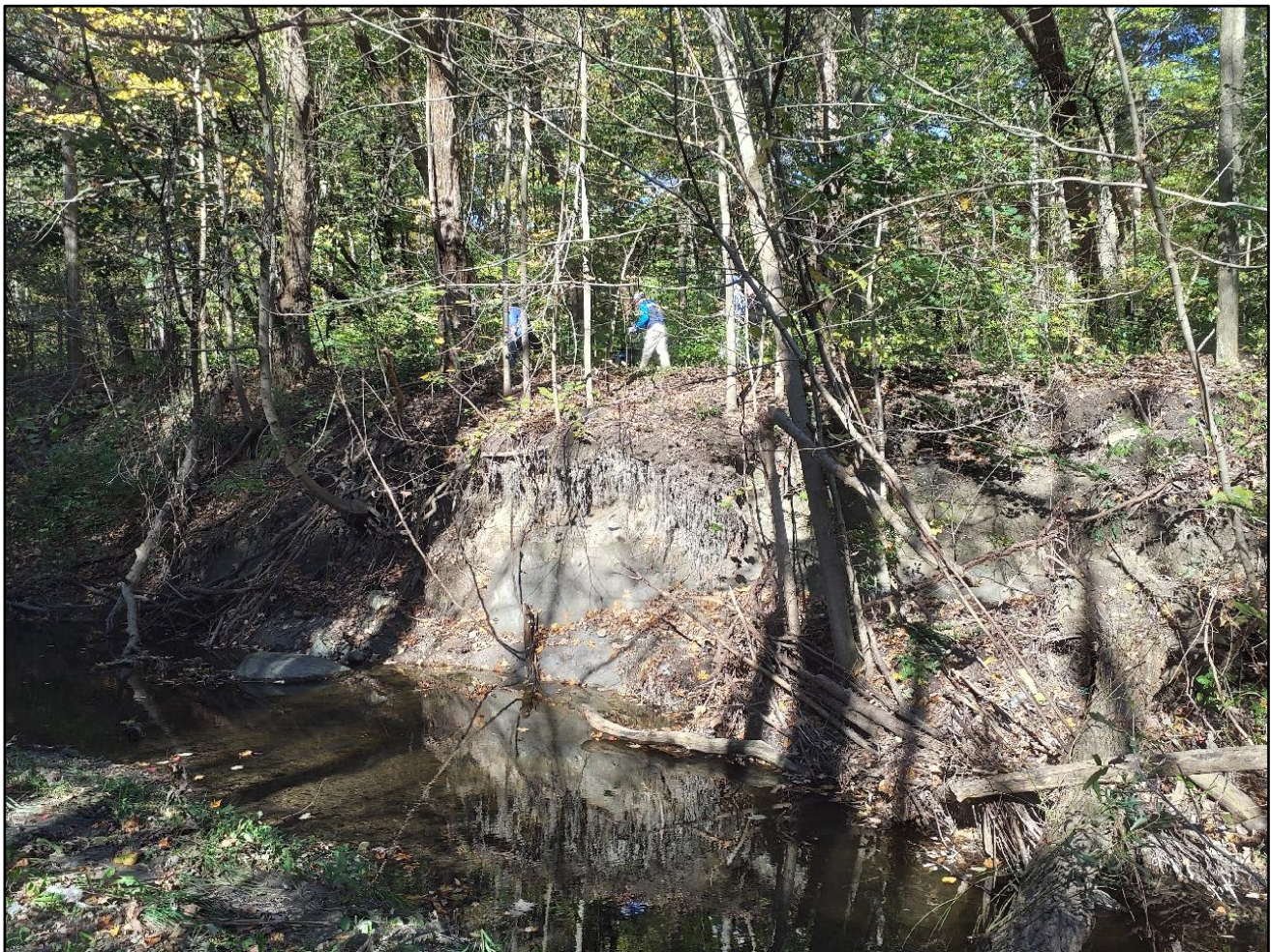
Figure 4-97: Degraded Channel Conditions at Priority Site #19. The Actively Eroding Bank has Created a Lateral Risk to a 675 mm diameter Sanitary Sewer
