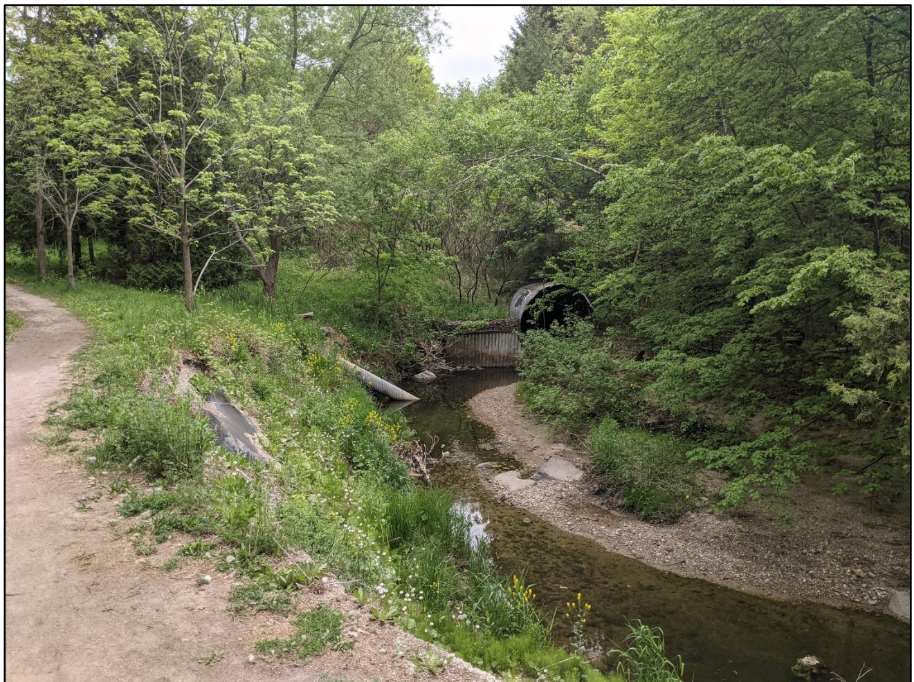
Figure 4-94: Degraded Channel Conditions at Priority Site #18. The Actively Eroding Bank has Created a Lateral Risk to a 675 mm Diameter Sanitary Sewer
