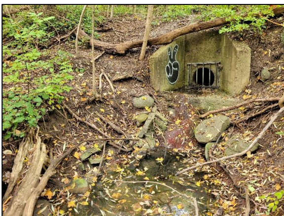
Figure 4-27: Northern Storm Sewer Outfall at Edge of Pedestrian Trail
