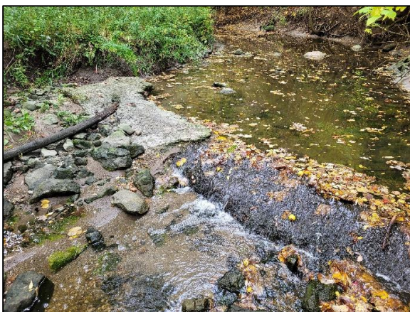
Figure 4-25: Exposed Concrete Encasement Surrounding 675 mm Ø Sanitary Trunk Sewer
