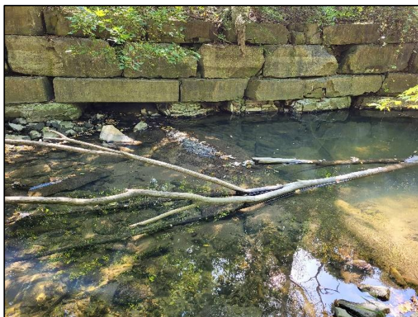
Figure 4-33: Exposed Encasement with Upstream Scour Pool
