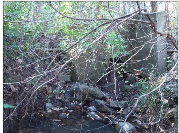
Figure 4-20: Eroded and Down-cut Outfall Channel Contributing to the Slumping of the Upstream Concrete Headwall Structure
