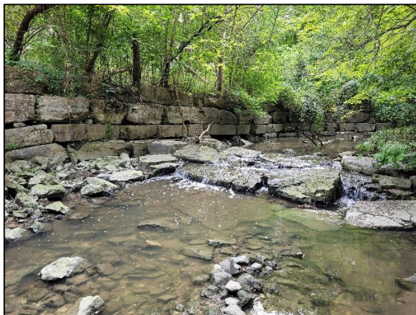
Figure 4-31: Armourstone Grade Control Structure and Armourstone Bank Protection
