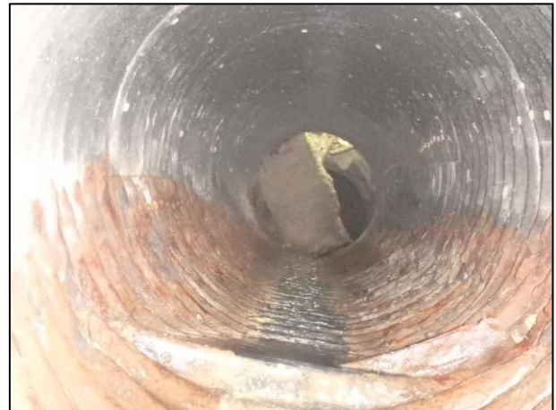
Figure 4-22: Obstructions and Detachments Within Upstream Pipe Segment
