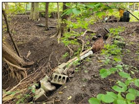
Figure 4-28: Southern Storm Sewer Outfall at Top of Slope and Associated Outfall Channel
