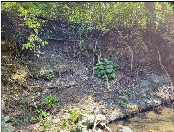
Figure 4-37: Erosion Scar Along Outer Bank Immediately Upstream of Exposed Sewer Encasement
