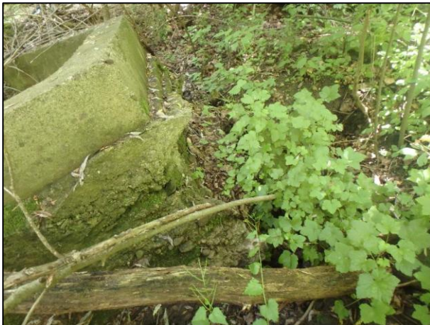
Figure 4-21: Detachment of Headwall From Inlet Pipe
