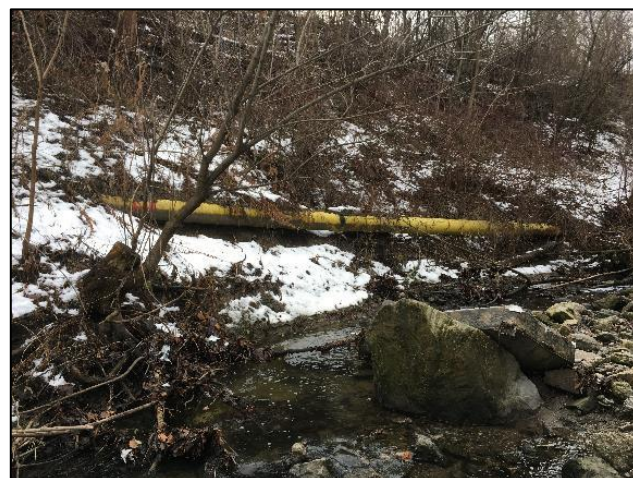
Figure 2-2: Photo of Sun-Canadian Pipeline Exposure in Bank of Newtonbrook Creek
