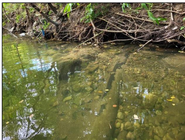
Figure 2-1: Photo of Trans-Northern Pipeline Exposure in Channel Bed of Newtonbrook Creek
