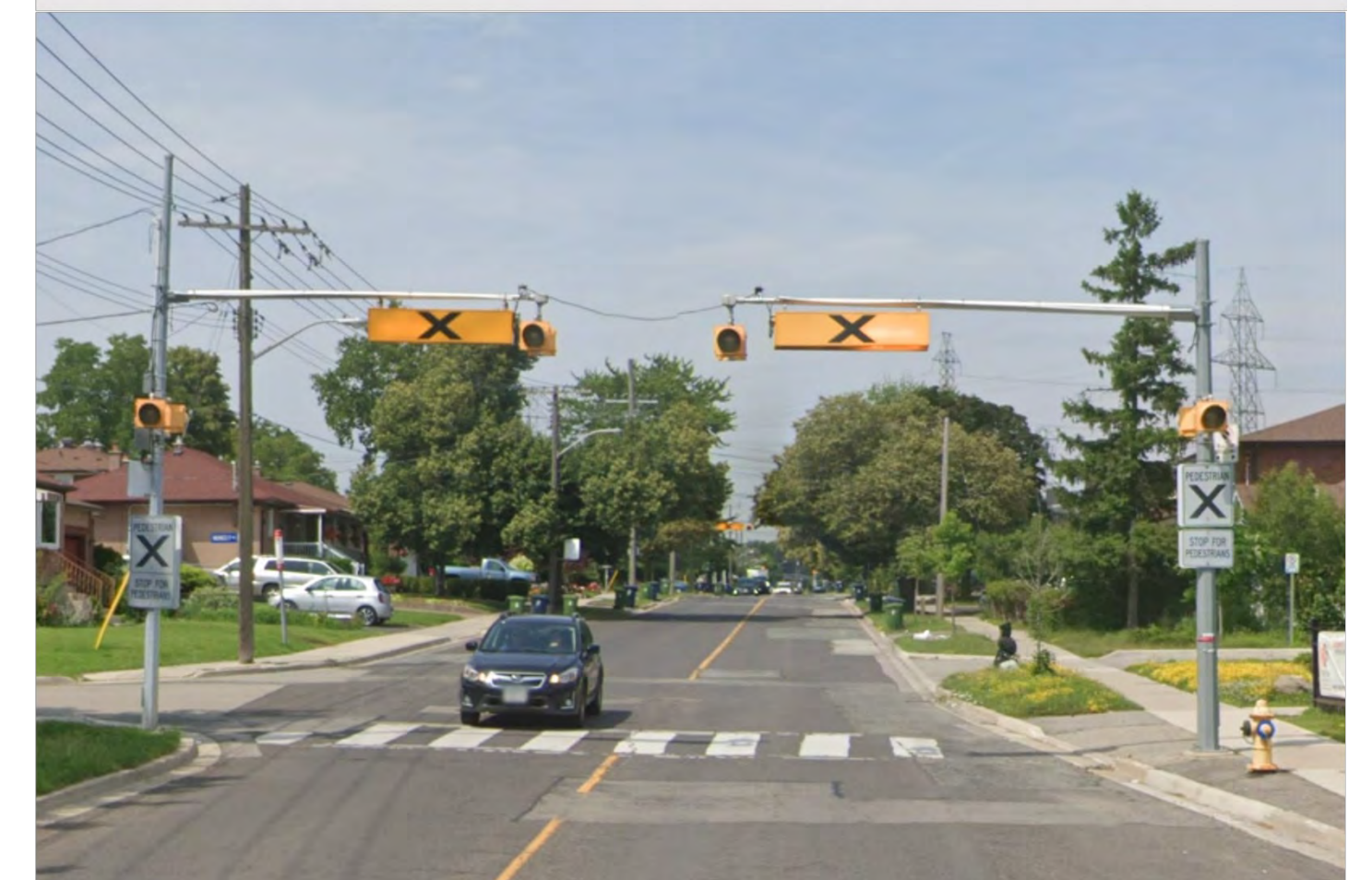
Crosswalk in School Area
