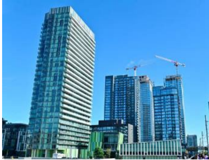
A tall multi-unit residential building
