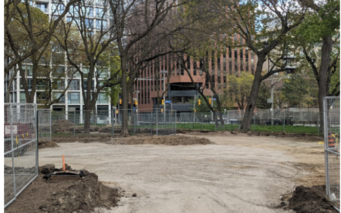
Figure 22: Preservation of mature trees during the construction of St. Andrew's Playground Park in Toronto by DTAH. Minimizing soil disruption and working with the existing canopy can have positive impacts on low carbon outcomes (DTAH, 2021).
