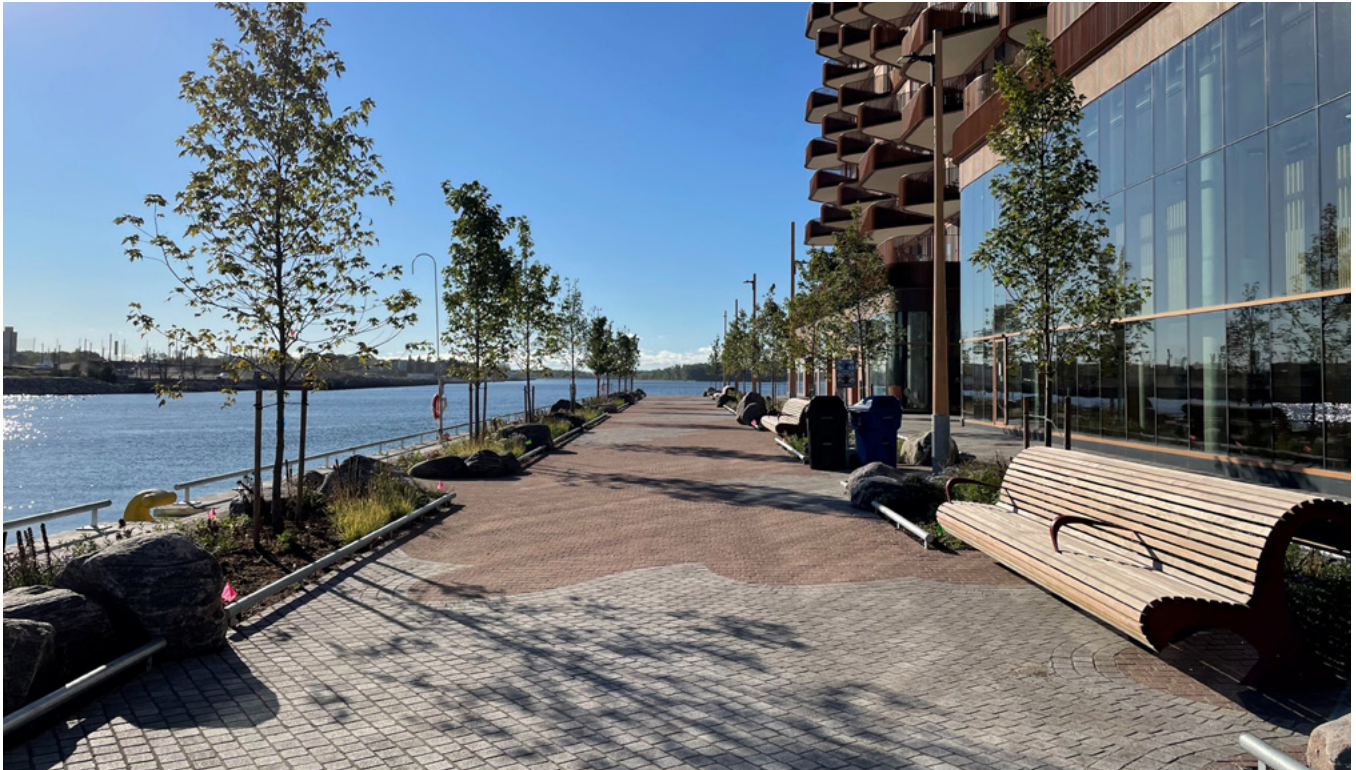
Figure 29: Open, shared tree planters at Toronto’s Water’s Edge Promenade provide continuous soil volume, aeration, and drainage that support stronger tree growth. Compared with hardscape-contained tree pits and soil cell systems, they can reduce concrete, edge restraint, and proprietary components, lowering material intensity and embodied carbon while improving constructability and maintenance access. (DTAH, 2025).
