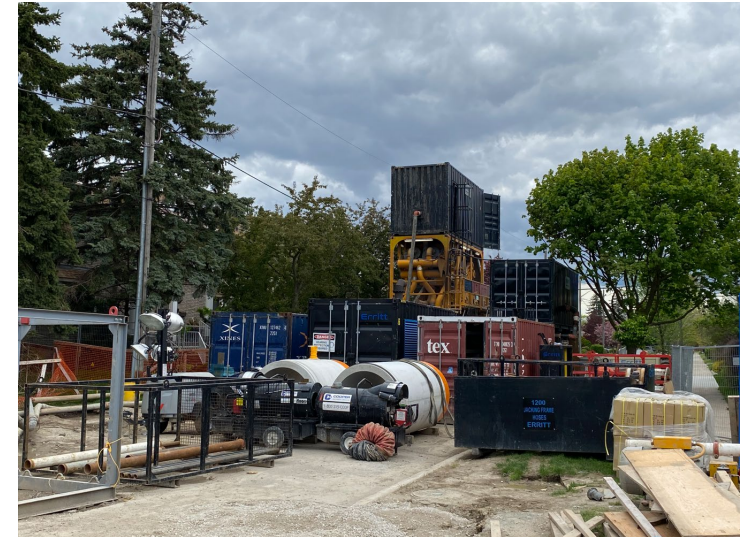
Support equipment at a tunneling site
