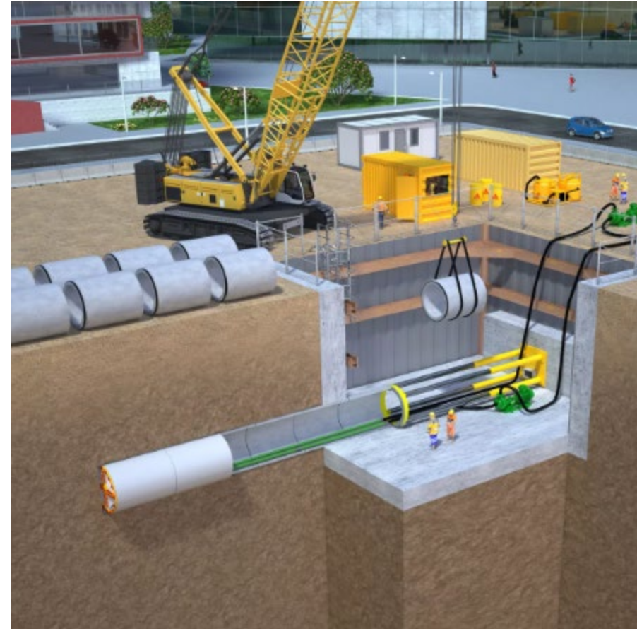
Image of microtunneling activities at a launch site
