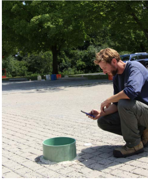
Figure 12: Surface infiltration testing conducted with a simple single-ring infiltrometer and a timer on the technician's mobile phone. Source: https://wiki.sustainabletechnologies.ca/wiki/Inspection_and_Maintenance:_Permeable_Pavement
