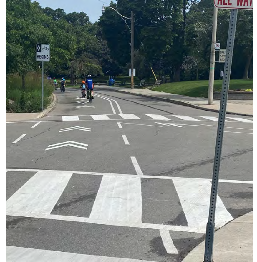
Intersection at Centre Rd. and Colborne Lodge Dr.
