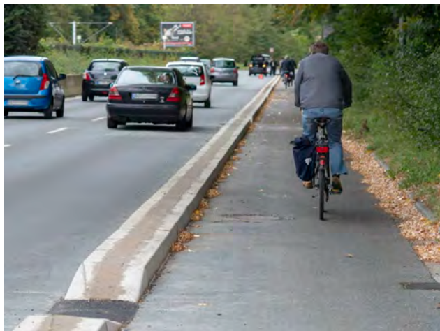
Protected Cycle Lane (Physical Barrier)
