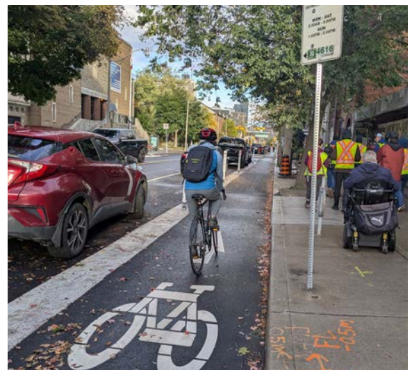
Cycle track upgrades on Harbord Street.
