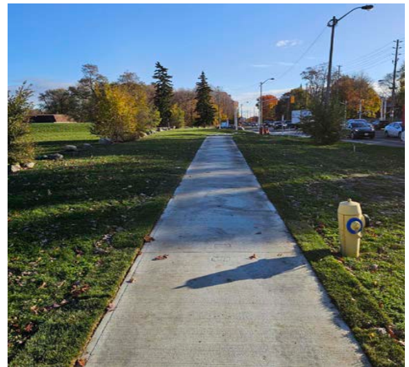
New sidewalk on Eglinton Avenue West at Wincott Drive
