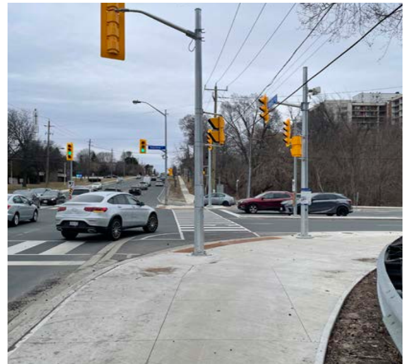
Truck Apron at Steeles Avenue East/Bayview Avenue
